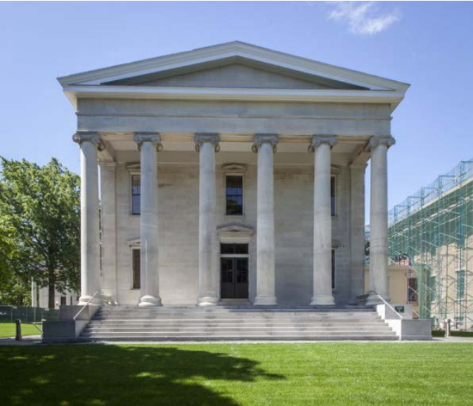
Snug Harbor Building E's exterior restoration
