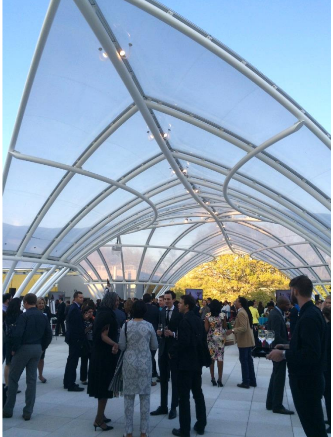
Brooklyn Children's Museum's new roof canopy
