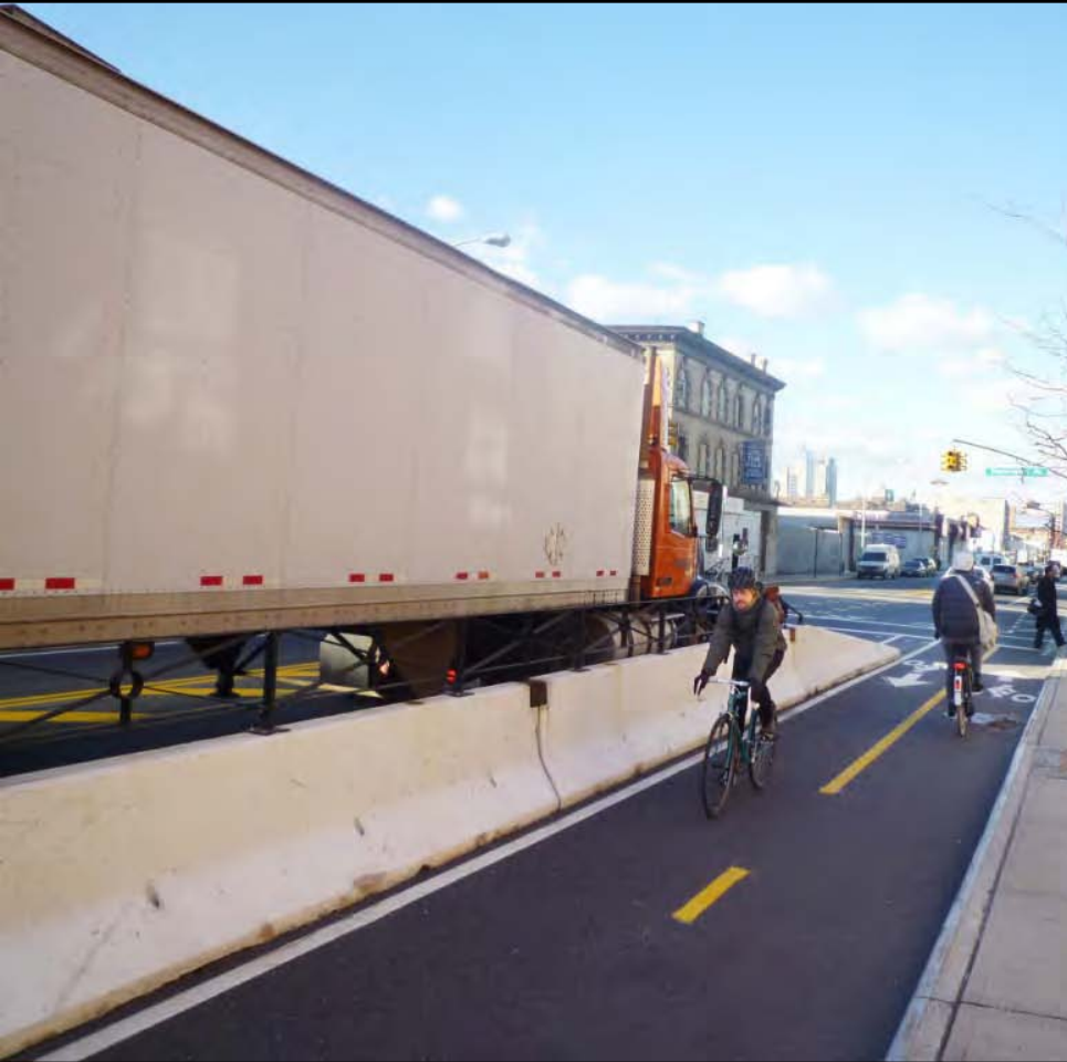
Flushing Ave, Brooklyn
