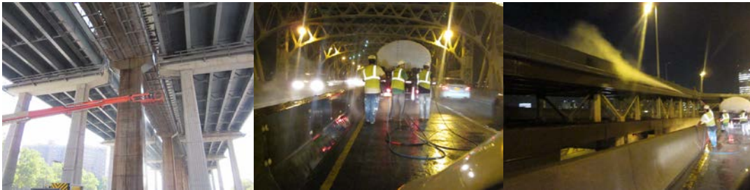
Washing the Williamsburg Bridge in July 2011 and the Ed Koch Queensboro Bridge in August 2011.
