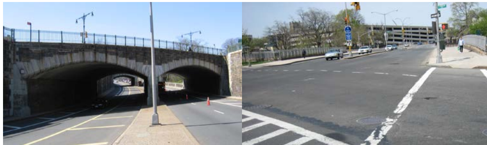
Southern Boulevard Bridge over East Fordham Road.
