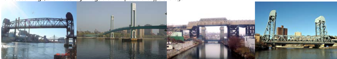
Lifted Roosevelt Island Bridge. (Credit: NYSDOT). Wards Island Pedestrian Bridge. Ninth Street Bridge. (9 th Street Credit: Bojidar Yanev) Broadway Bridge. (Credit: Bernard Ente)
