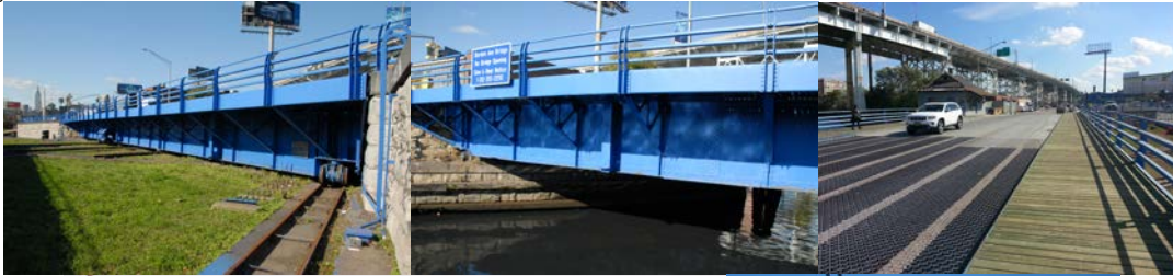
Borden Avenue Bridge. (1 st and 2 nd Credit: Peter Basich, 3 rd : Vadim Sokolovsky Carroll Street Bridge. (1 st Credit: NYSDOT, 2 nd : Russell Holcomb)
