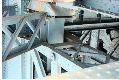
Truss Bearing on Manhattan Bridge. (Credit: NYSDOT)
