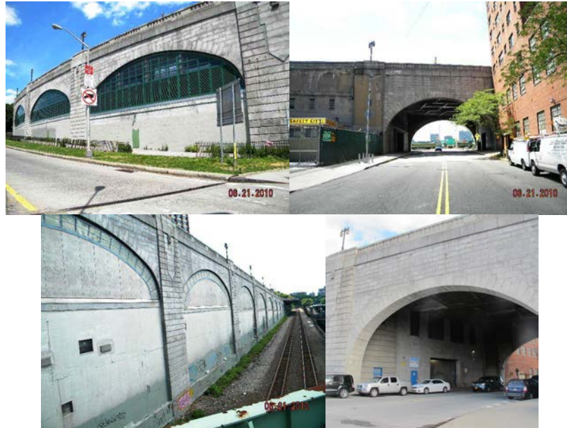
Riverside Drive Bridge in 2010. (Credit: NYSDOT) Vehicle Repair Facility.
