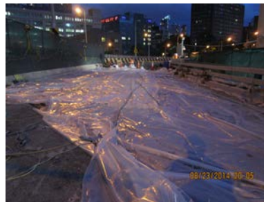
August 2014: Brooklyn-Bound Sands Street Structure Curing After Closure Pour Concrete Placement.
