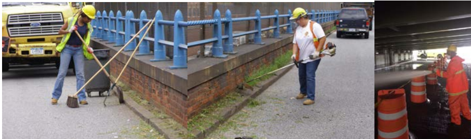
Assistant City Highway Repairer Lashawn Elam and Highway Repairer Anita Ramos Removing Vegetation and Other Debris. Assistant City Highway Repairer E'boni Brown Removing Debris under the Henry Hudson Parkway at 58 th Street. (HHP Credit: Edward Pedersen)
