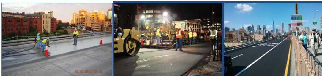
October 2014: Brooklyn-Bound Approach Waterproofing.
