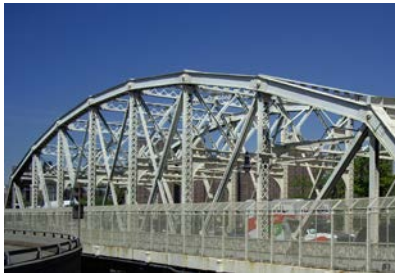
Macombs Dam Camelback Truss.
