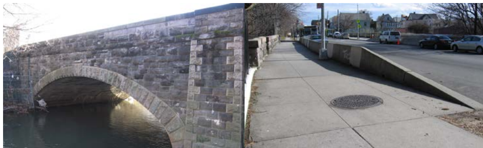
East 180 th Street Bridge over Bronx River.
