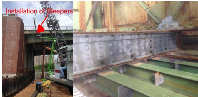
Hutchinson River Parkway Bridge - Installation of Sleeper Steel Beams to Directly Support the Steel Grating.
