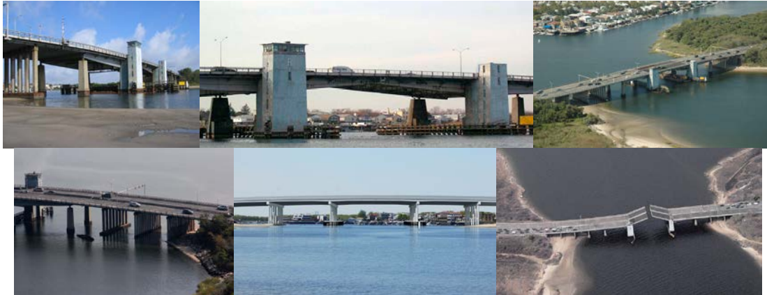
Current Belt Parkway Bridge Over Mill Basin. Aerial Views. Proposed Bridge. Open Bridge.
