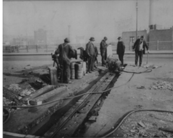
Constructing an Expansion Joint on the Riverside Drive Viaduct in 1918.
