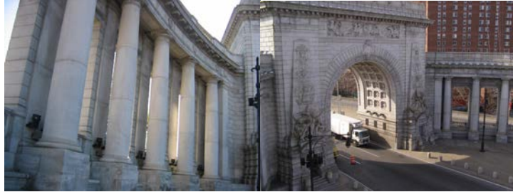
Manhattan Bridge Colonnade. (Credit: Peter Basich) Arch and Part of the Colonnades in March 2011. (Credit: Bojidar Yanev)
