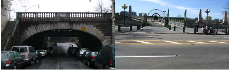
Riverside Drive Bridge over West 138 th Street.
