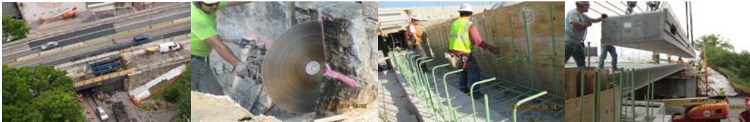
June 2014: Stage II Deck Removal of Westbound Bridge Deck. Veteran's Memorial Pier at Top. July 2014: Saw Cutting the Existing Northwest Abutment. Setting Rebars at the Northwest Abutment. August 2014: Lowering the Last of the Seven Pre-cast Concrete Box Beams on the North Side Abutments.
