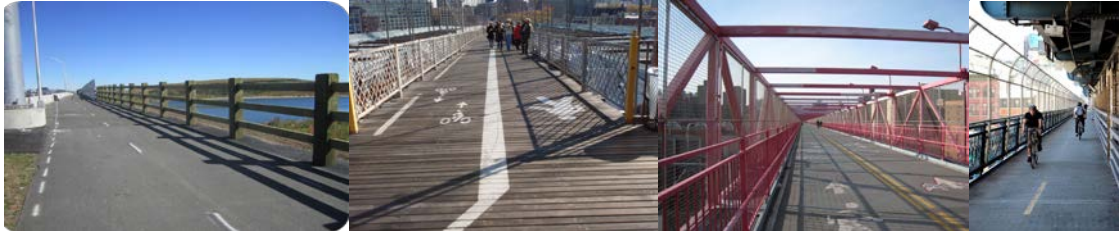
Fresh Creek Bicycle/Pedestrian Path in 2013. Brooklyn Bridge and Williamsburg Bridge Bicycle/Pedestrian Paths in 2010. (Williamsburg Credit: Russell Holcomb) Manhattan Bridge Bicycle Path in 2013.
