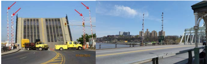
Metropolitan Avenue Bridge over English Kills Warning Gates. (Credit: NYSDOT) West 207 th Street/West Fordham Road Bridge Warning Gate.
