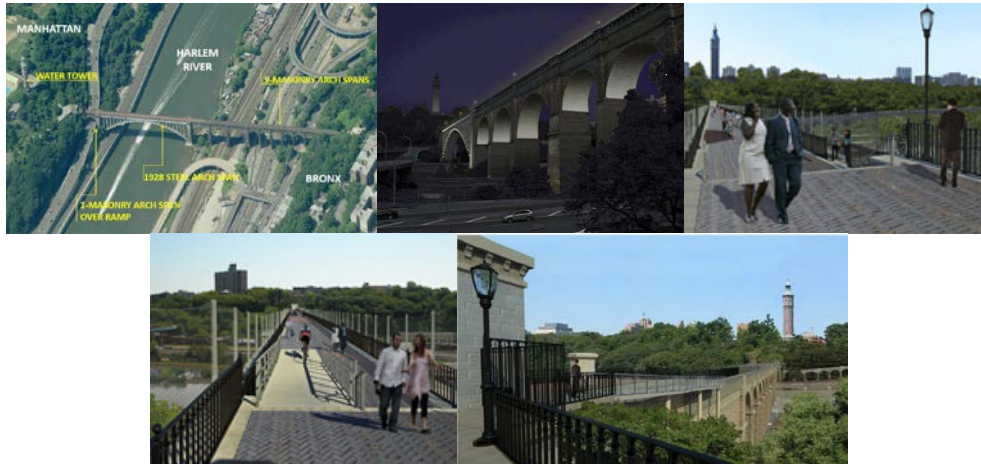
Project Overview. Rendering of the Restored High Bridge, View From the Bronx to Manhattan, View From Manhattan to the Bronx, and ADA Access Area.
