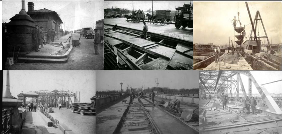
Willis Avenue Bridge Curbing and Road Repair in the Early 1920's. Madison Avenue Bridge Center Pier Under Construction in September 1909, and Constructing New Guardrail in September 1934. City Island Bridge Concreting in 1912. University Heights Bridge Roadway Repair in 1923.
