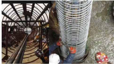
City Island and Gerittsen Inlet Bridge Rebar Cages.
