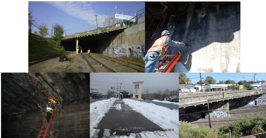
Metropolitan Avenue Bridge in 2009. (Credit: NYSDOT) 2010 Inspection - Hands-On Inspection of A Pier. Obtaining a Steel Coupon Sample From a Stringer. February 2014: View of Plates on Left Sidewalk (Fresh Pond Road). September 2014: Spans 1 and 2 Right Concrete Parapet. (Parapet Credit: NYSDOT)
