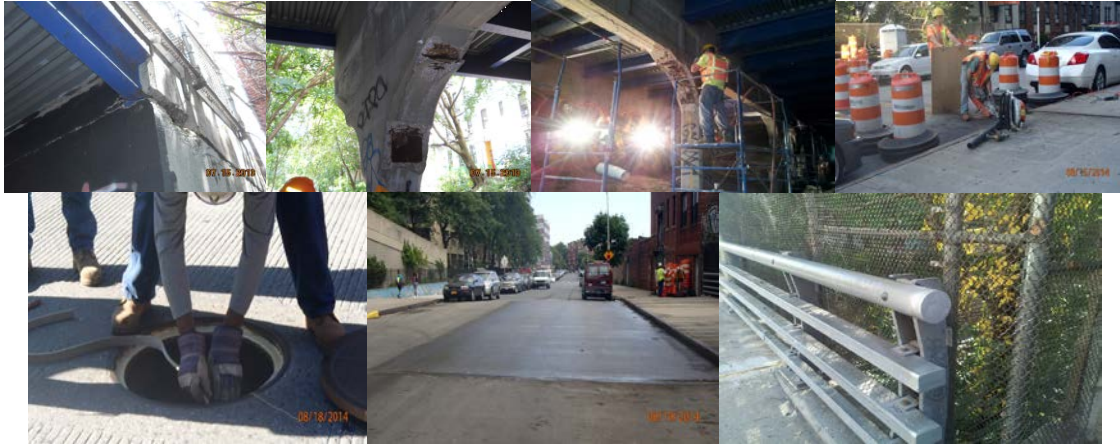
Crown Street Bridge Before, During, and After Construction.
