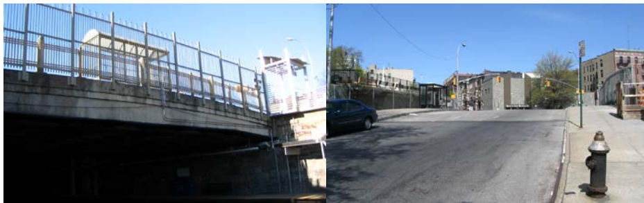
East 162 nd Street Bridge over MNRR.
