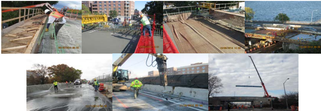
June 2014: Stage II Deck Removal of Westbound Bridge Deck. Veteran's Memorial Pier at Top. July 2014: Saw Cutting the Existing Northwest Abutment. Setting Rebars at the Northwest Abutment. August 2014: Lowering the Last of the Seven Pre-cast Concrete Box Beams on the North Side Abutments.
