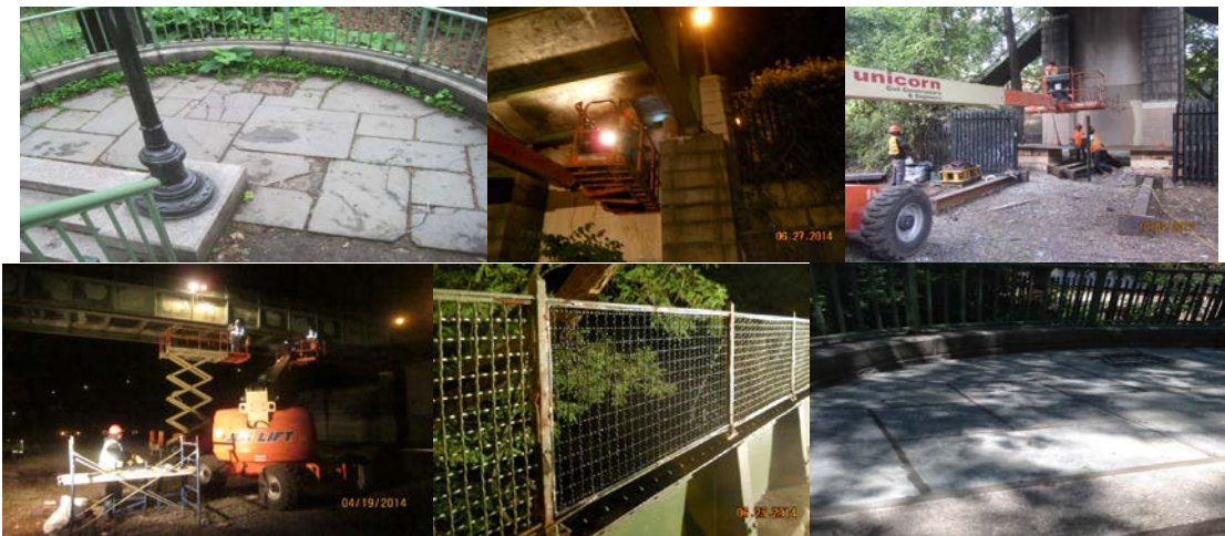
West 148 th Street Bridge Before, During, and After Construction.
