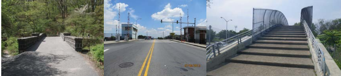
End Approach to Bridge Over Dam at Clove Lake. Metropolitan Avenue Bridge Approach. (Metropolitan Credit: NYSDOT) Belt Parkway Bridge over 26 th Avenue Approach. (Credit: Artemio Angeles)
