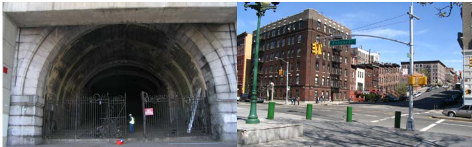
Riverside Drive Bridge over West 145 th Street.
