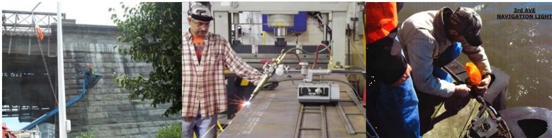
Cleaning the Brooklyn Bridge Brooklyn Anchorage in July 2007. (Credit: Serag Saad) Bridge Repairer and Riveter James Philip Using a Track-Mounted Torch to Bevel the Edge of a Steel Plate in September 2012. (Credit: Thomas Whitehouse) Checking the Navigation Lights at Pier #5 of the Third Avenue Bridge.
