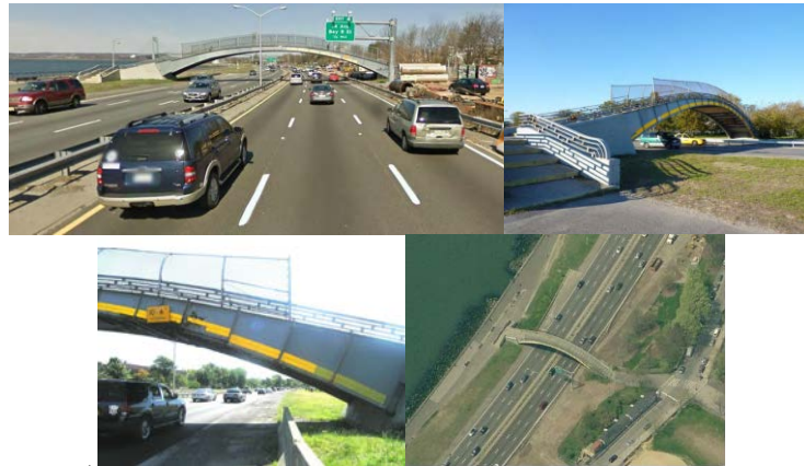
17 th Avenue Bridge – Existing Conditions. Deteriorated Left Girder.
