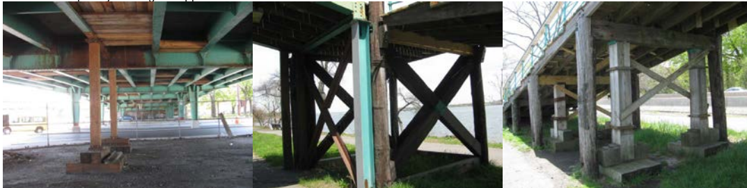
2014: Timber Shoring at Spans 7 and 8 of the Harlem River Drive over Ramp to and From Northbound Harlem River Drive. Steel Shoring of the Damaged Column at Pier 4 of the Crocheron Park Pedestrian Bridge. Timber Shoring at Piers 5 and 6.
