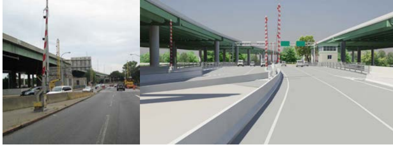
Looking East – Towards Current And Proposed Bridge.
