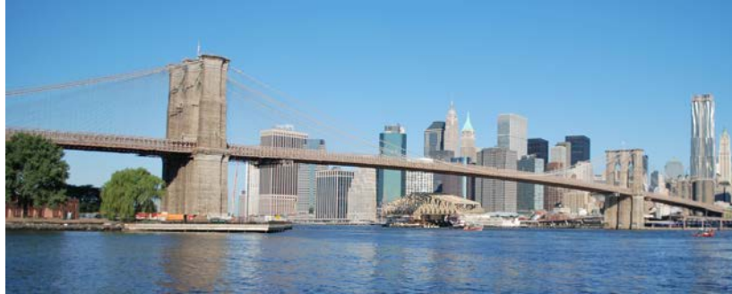
Voyage up the East River on July 26, 2010. New Willis Avenue Bridge Span Passing Under the Brooklyn Bridge. (Credit: Douglas Reese)
