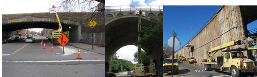
Inspecting the Belt Parkway Bridge over 26 th Avenue in December 2012. (Credit: Artemio Angeles) Inspecting the Nereid Avenue Bridge over Bronx River Parkway in June 2012, Using a 60 Foot Boom With Outriggers. (Credit: Bojidar Yanev) Inspecting the Brooklyn-Queens Expressway (Eastbound) over Cadman Plaza/Brooklyn-Queens Expressway (Westbound).
