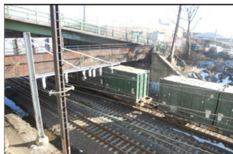
Bryant Avenue Bridge in 2011. (Credit: NYSDOT)
