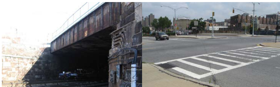
East 165 th Street Bridge over MNRR.
