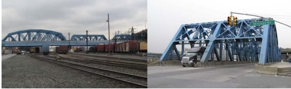
Leggett Avenue Bridge over Amtrak.
