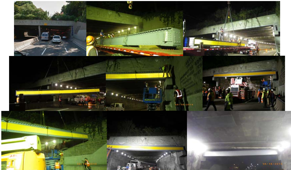
FDR Drive Structure. Installation of the Protection Beam.
