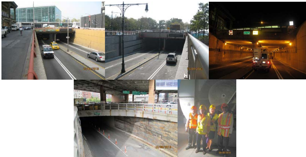
October 2013 – Battery Park Underpass – Elevation Right Span 1 and Left Span 1. (Credit: NYSDOT) September 2013 - Span 2 Looking Westbound (FDR Drive to West Street) West Street Underpass - Elevation Right Span. (Credit: NYSDOT) September 2014: Project Team in the Battery Park Underpass – Mechanical Engineer Bidyut Niyogi, Construction Project Manager Beatriz Duran, Project Manager Tamara Berlyavsky and Administrative Engineer Bhaskar Gusani.
