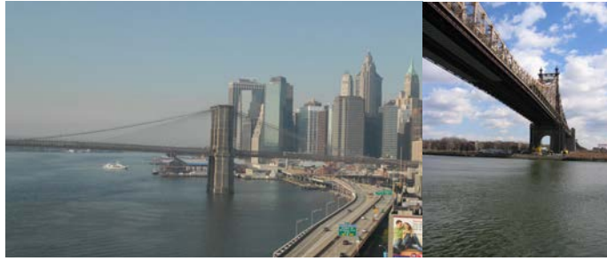
Brooklyn Bridge in 2009. (Credit: Jagtar Khinda) Ed Koch Queensboro Bridge in 2006. (Credit: Russell Holcomb)
