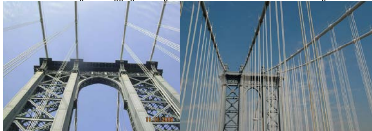
Manhattan Bridge Suspenders. (Credit: NYSDOT and Jagtar Khinda)
