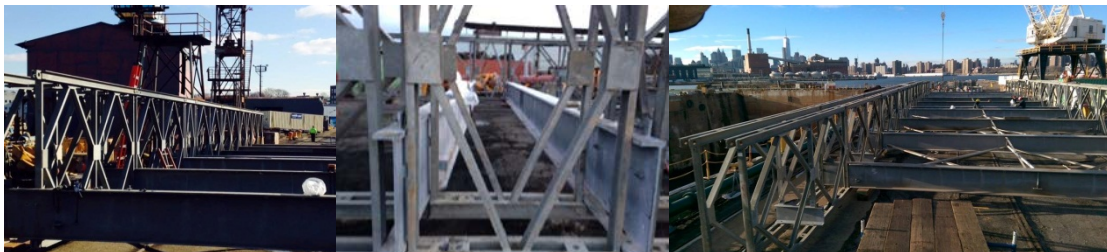
The Contractor Assembled the Temporary Bridge Segments at the Brooklyn Navy Yard. The Pieces Were Transported to City Island by Barge.
