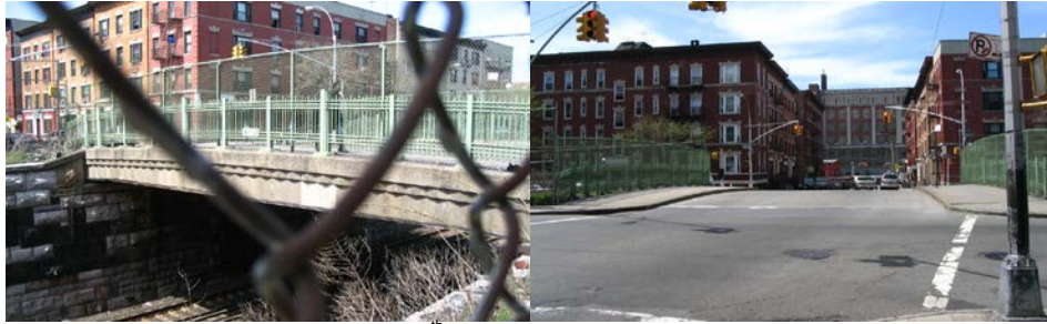
East 187 th Street Bridge over MNRR.
