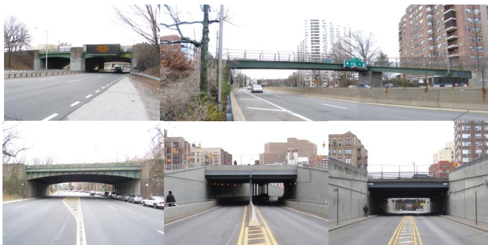
East Tremont Avenue Bridge over Hutchinson River Parkway, 236 th Street Pedestrian Bridge over Henry Hudson Parkway, Henry Hudson Parkway Bridge over Broadway, Grand Concourse Bridge over Burnside Avenue, and Grand Concourse Bridge over East 204 th Street.
