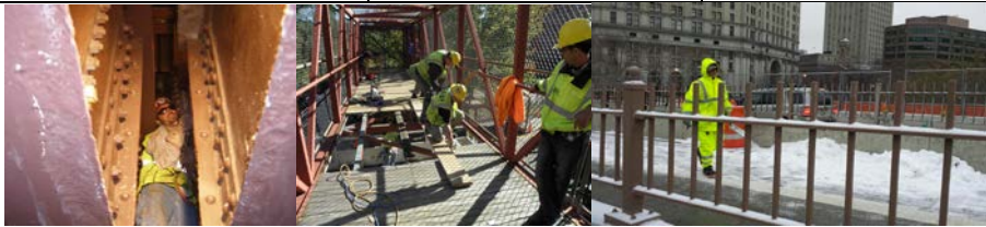
Bridge Repairer Riveter Damian Venezia Squeezing Between the Girders to Access a Floor Beam That Needed to be Reinforced on the Ed Koch Queensboro Bridge – August 2010. (Credit: Hany Soliman) Carpenters John Horgan and Ruben Urena, and Assistant Civil Engineer Fouad Althaibani Repairing the PS-5 Bridge in November 2011. (Credit: Thomas Whitehouse) Cement Mason Victor Porowski Spreading Sodium Acetate on the Walkway of the Brooklyn Bridge in 2013. (Credit: Paul Schwartz).
