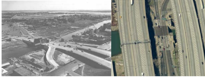
Unionport Bridge in 1953 and 2009.
