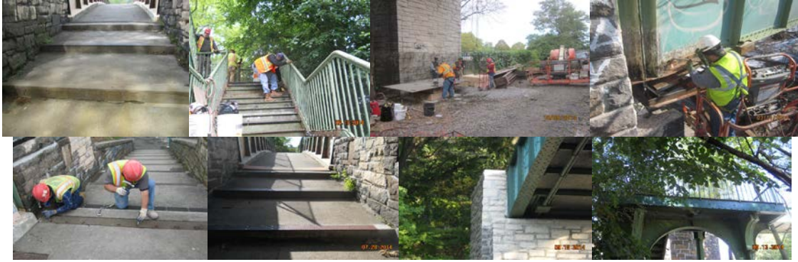
Inwood Hill Park Footbridge Before, During, and After Construction.
