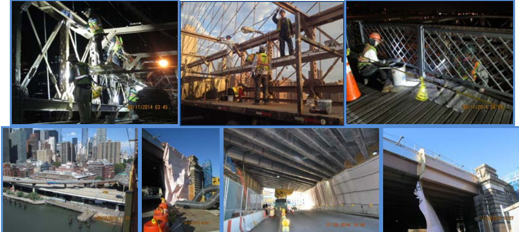
August 2014: Main Bridge Touch-Up Painting, and Painting Manhattan Main Span Promenade Railing. August 2014: Painted Manhattan Ramps. October and November 2014: Blasting and Painting – Brooklyn Approach Structures.
