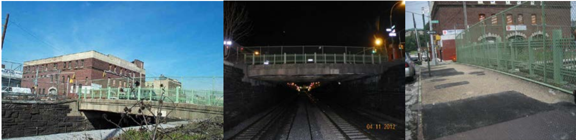
East 175 th Street Bridge in 2002 and 2012. (Credit: NYSDOT) South Sidewalk.
