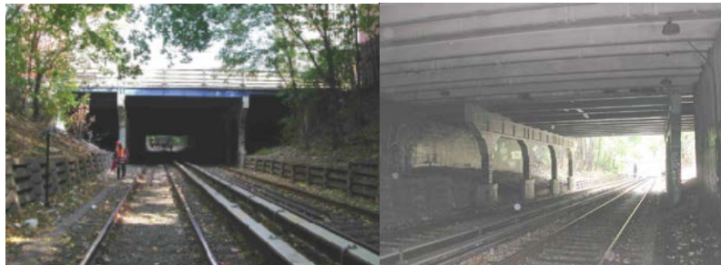
Crown Street Bridge. Right Elevation in 2011. (2011 Credit: NYSDOT)
