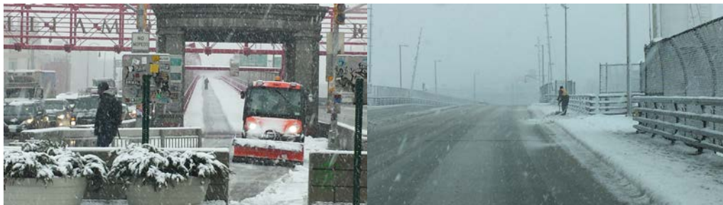
February 3, 2014: Cement Mason Luigi Mula Operating Snow Clearing Equipment on the Williamsburg Bridge. Bridge Operator Shoveling Snow on the Greenpoint Avenue Bridge. (Credit: Paul Schwartz)
