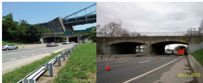
4th Avenue Bridge. March 2010: Right Elevation. (Credit: NYSDOT)
