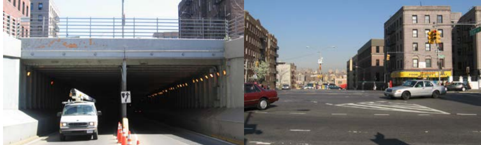
Grand Concourse Bridge over East 167 th Street.
