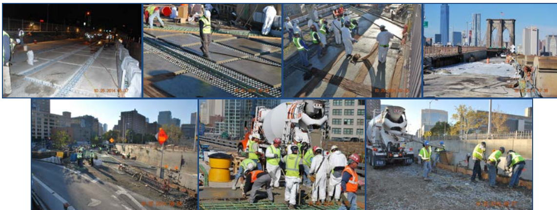
October 2014: York Street Structure – Closure Pour. Sands Street Structure – Curb Mall.
