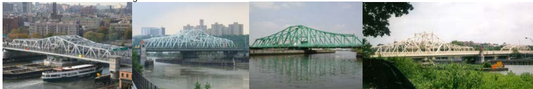
Third Avenue and University Heights Bridges. (Credit: Michele N. Vulcan) Grand Street Bridge. (Credit: NYSDOT) Macombs Dam Bridge. (Credit: Michele N. Vulcan)
