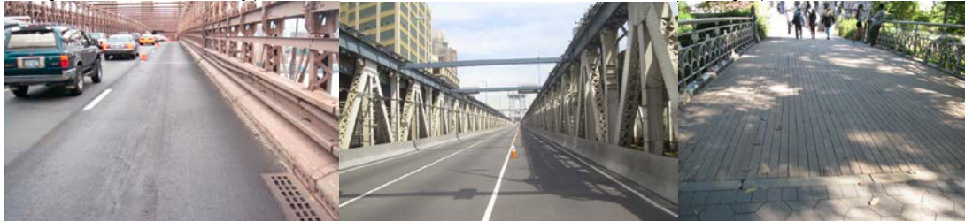
Brooklyn Bridge Wearing Surface. Manhattan Bridge Wearing Surface and Safety-Shaped Barriers. (Credit: NYSDOT) West 86 th Street Pedestrian Bridge (Southwest Reservoir Bridge) Wooden Wearing Surface.
