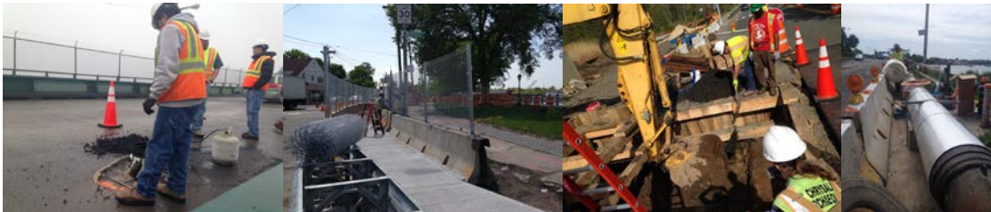
February 2014: Pothole Repair. August 2014: Contractor Constructing a 5-Foot Wide Walkway to Protect and Guide Pedestrians Around the Designated Work Zone on the Esplanade. Excavating on the West Side of the Bridge in the Presence of an Archeologist. Insulating the Temporary Water Main to Protect Against Low Temperatures and Accidental Impact.
