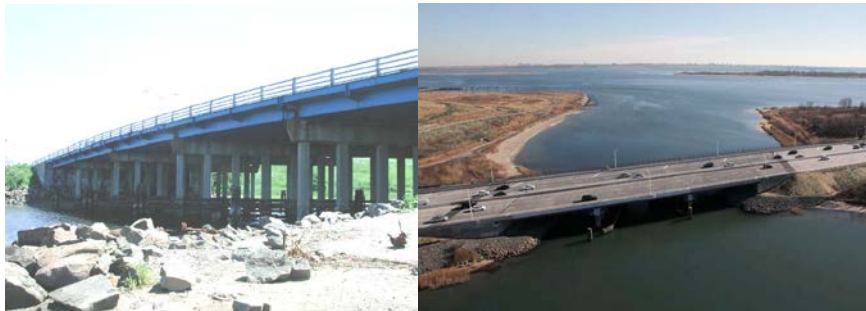
Old Fresh Creek Bridge. New Bridge in November 2013. (2002 Credit: NYSDOT)
