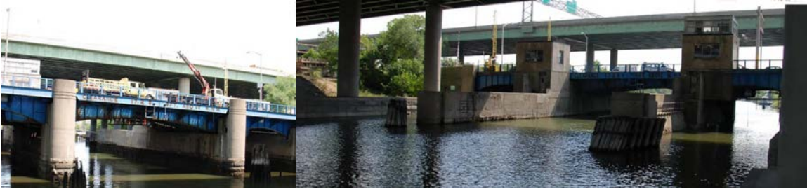
Existing Bridge - Looking North. Looking South.
