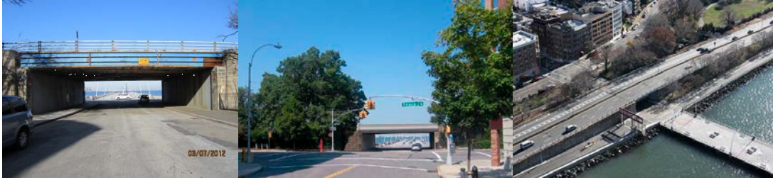
Bay Ridge Avenue Bridge in 2012. (Credit: NYSDOT) Proposed Bay Ridge Avenue Bridge. Current Aerial View.
