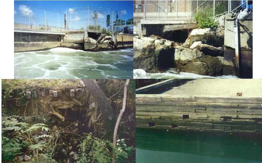
From Study of FDR Drive: Location #2 – Damaged Seawall at Segment #5. Sinkhole at Location #6 at East 59 th Street. From Study of Carroll Street Bridge: General View of the Southwest Crib Wall With the Delamination of the Timber Stretchers in the Tidal Zone.
