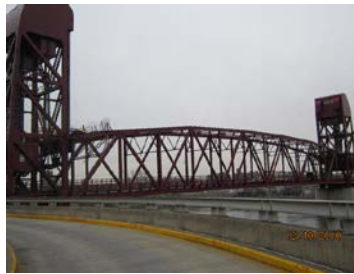
Elevation View of Roosevelt Island Bridge. (Credit: NYSDOT)
