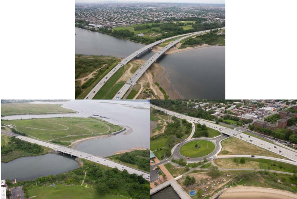
Summer 2014: Paerdegat, Fresh Creek, and Rockaway Parkway Bridges.
