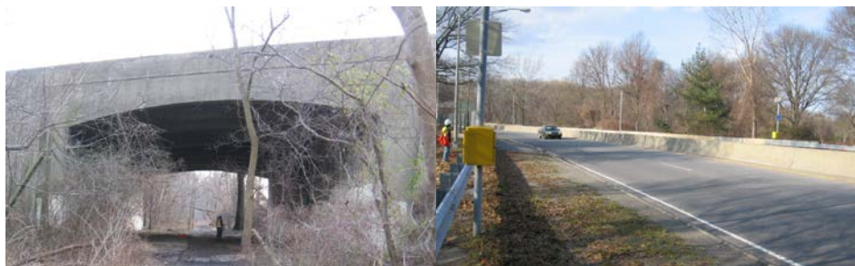
Mosholu Parkway Bridge over Conrail (Abandoned).
