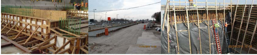
West 252 nd Street Bridge Formwork at the Pier and West Abutment in 2007. Formwork for the Westbound Roadway of the Rockaway Parkway Bridge in 2010. (Rockaway Bridge Credit: Eric Callender) Gerittsen Inlet Bridge in March 2014: Putting up Insulated Forms in Preparation for the Placement of Concrete at the West Abutment Wingwall. The Insulation Helps Protect the Concrete From the Elements and Fluctuating Temperatures During the Curing Period.
