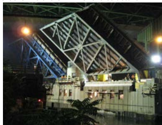
Leaves of the Hamilton Avenue Bridge.
