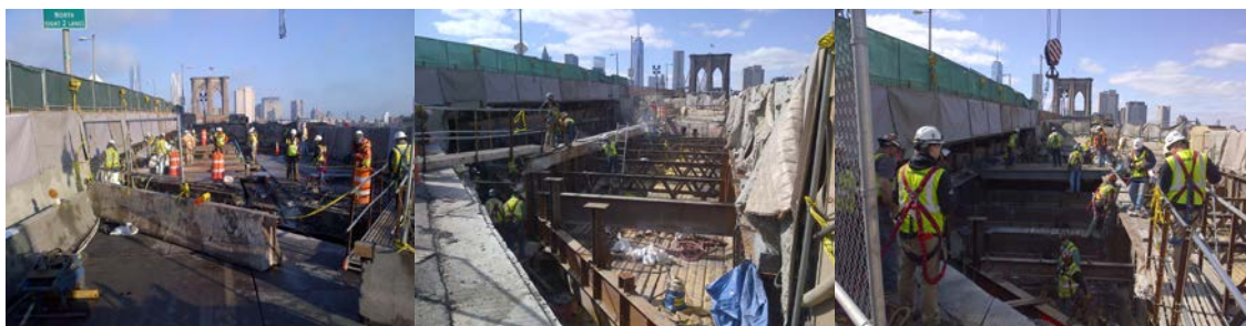
April 2014: Saw Cutting of the York Street Deck.
