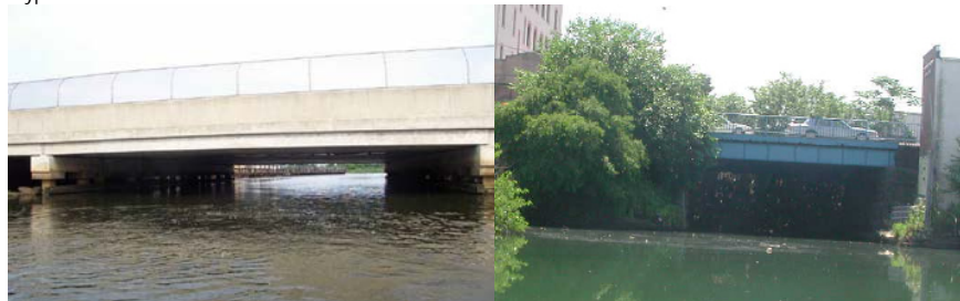
Hook Creek Bridge and Brooklyn's Third Avenue Bridge. (Credit: NYSDOT)
