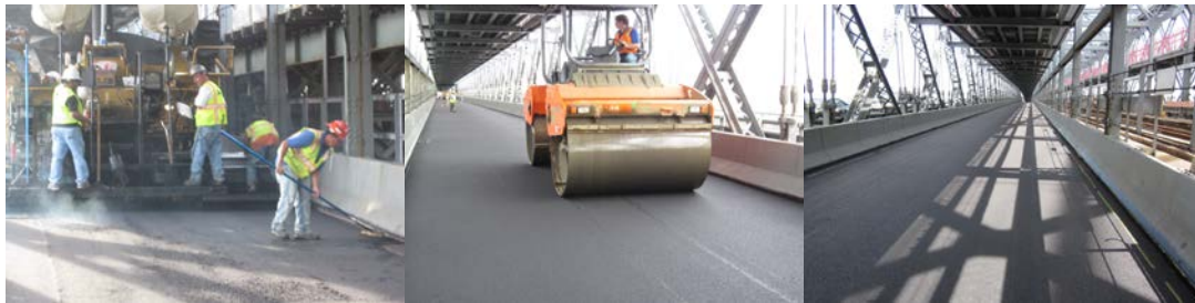
Repaving the Williamsburg Bridge in 2011.
