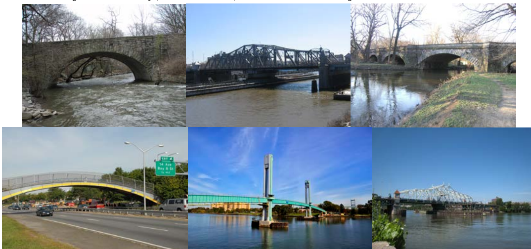
Southern Boulevard, Madison Avenue, and Moshulu Parkway Bridges. (Credit: Russell Holcomb) 17 th Avenue Pedestrian Bridge. (Credit: Peter Basic) Wards Island Pedestrian Bridge in October 2011. (Credit: Rafael Lopez) University Heights Bridge in July 2011. (Credit: Russell Holcomb)
