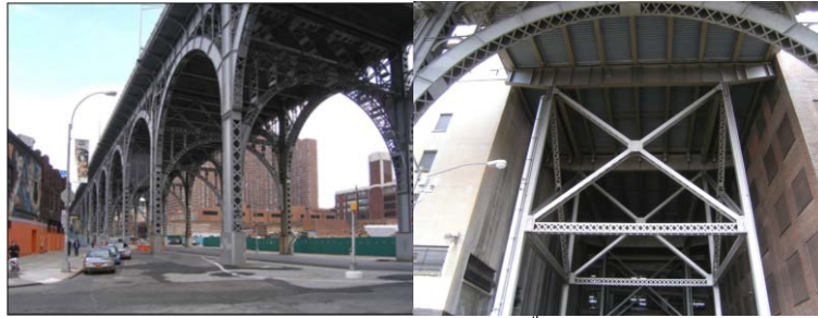
Riverside Drive Viaduct and West 134 th Street Bridge.
