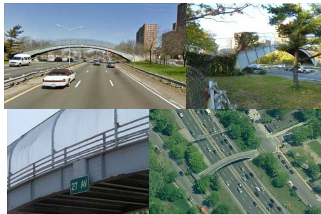
27 th Avenue Bridge – Existing Conditions.
