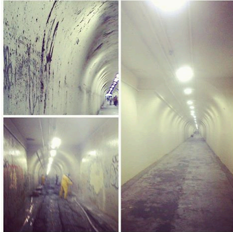
West 191 st Street Tunnel - Before and After.
