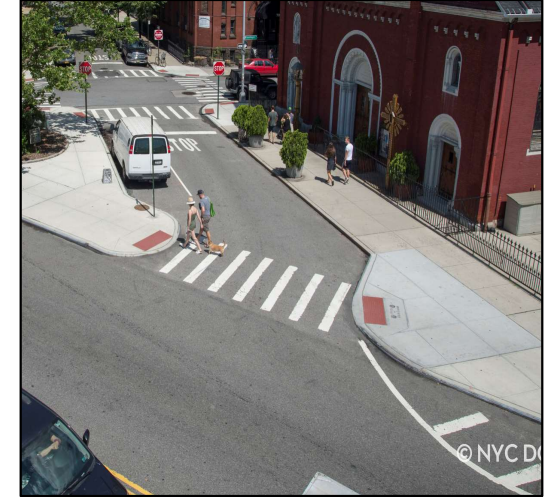
Concrete Curb Extensions
