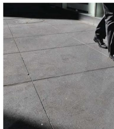
**PIGMENTED CONCRETE WITH SILICON CARBIDE TREATMENT 5FTX5FT SCORING**
