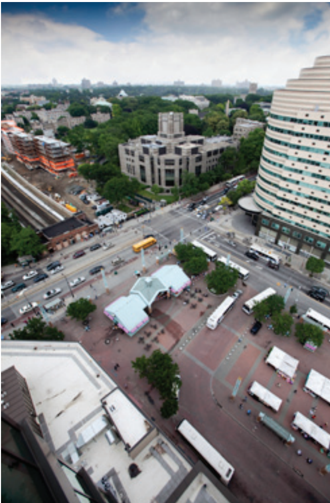
View towards northeast from Fordham Place (Existing)
