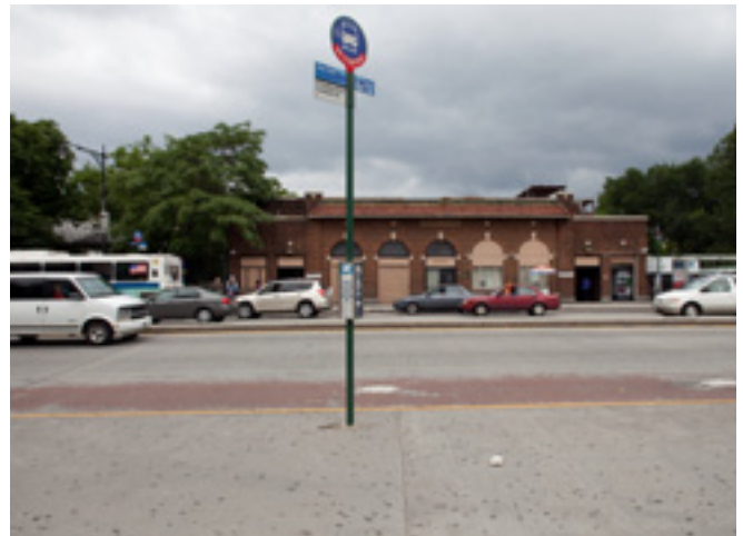
View from south side of Fordham Rd to historic Fordham MNR Station
