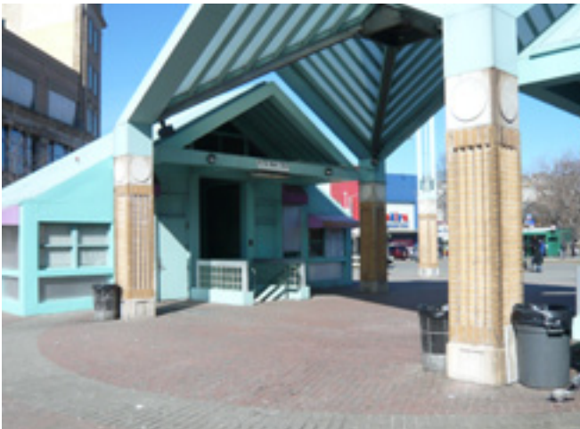
MNR station stair entry at Plaza
