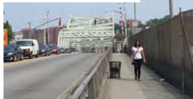
2A. University Heights Bridge, existing path
