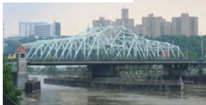
University Heights Bridge
