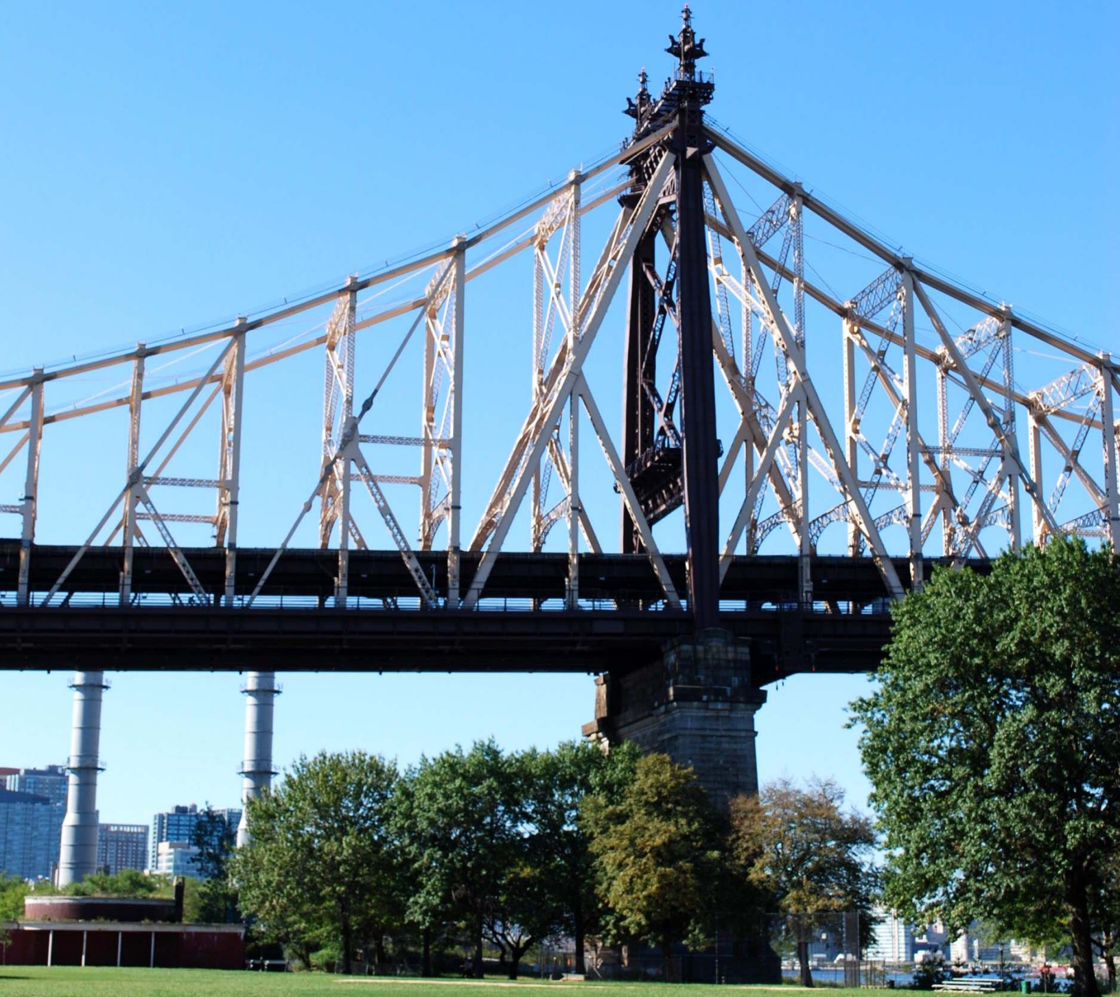
Ed Koch Queensboro Bridge over the East River between Manhattan and Queens
