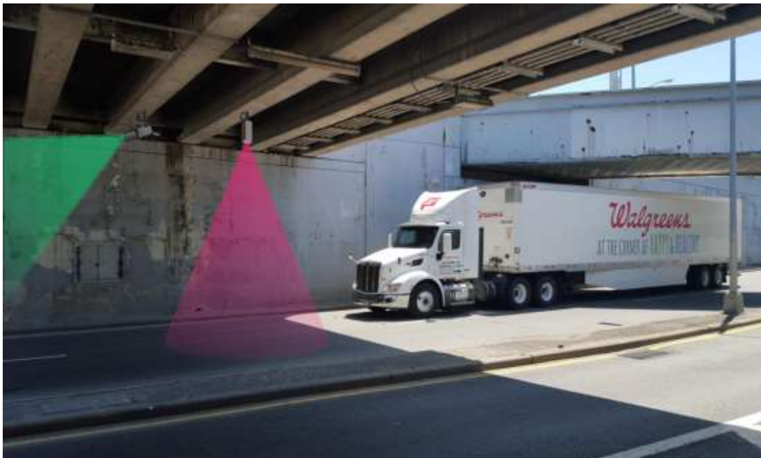
Typical laser detector installation
