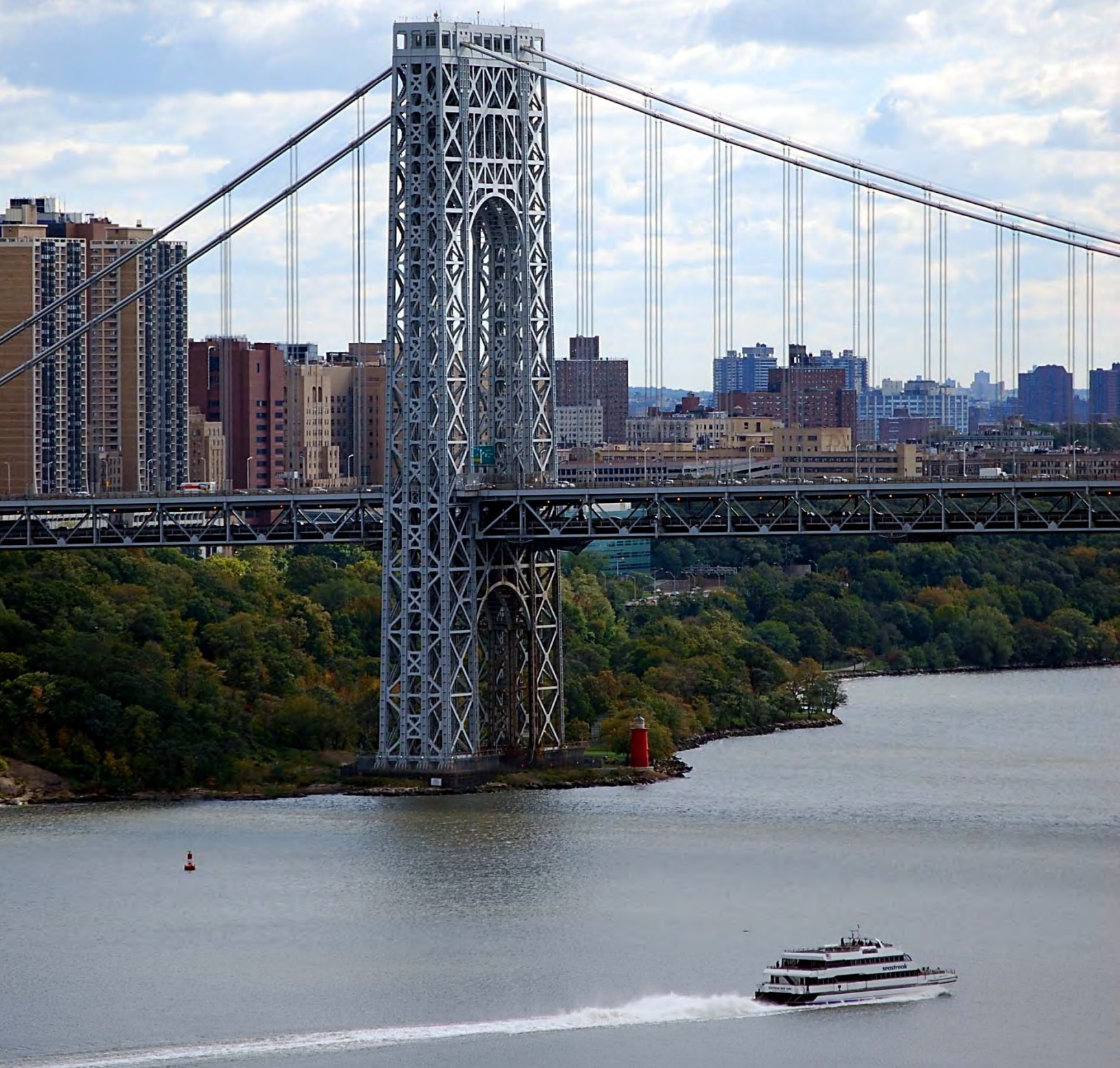
George Washington Bridge
