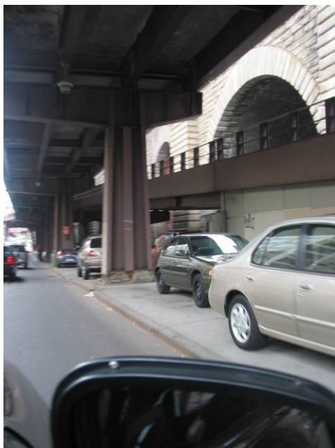
Figure 44 - Sidewalk Parking under Brooklyn Bridge
