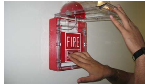
Activate a double action station
