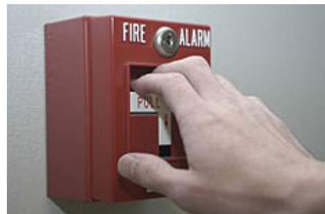
Activate a single action station
