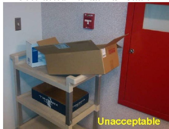
Obstructed Manual Pull Station
