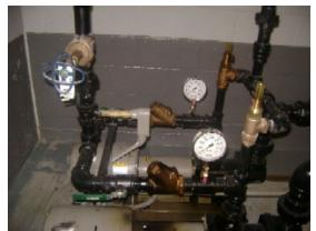
Pump connected to piping with the pressure gauge and control valves
