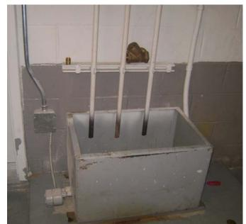
"Overflow catch Basin" or Tank with attached leak detection alarm
