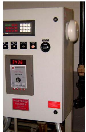
Working indicator with audible alarm attached; DIAGRAM
