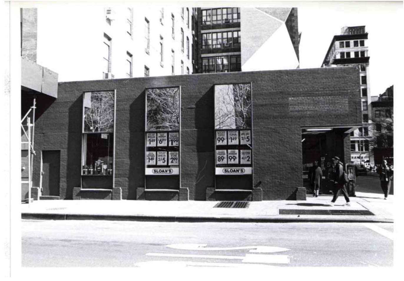
Photo at Mercer Street Facade
