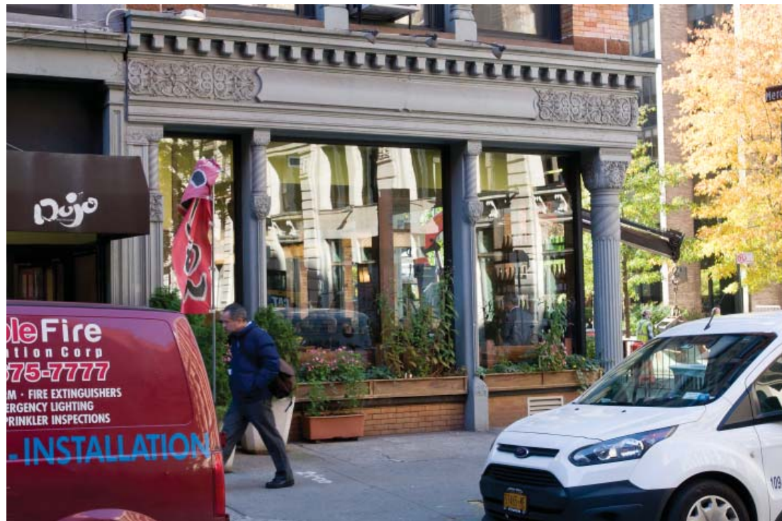
photo 3: 258 Mercer Street - Southeast Corner Mercer & West 4th (1894-95)
