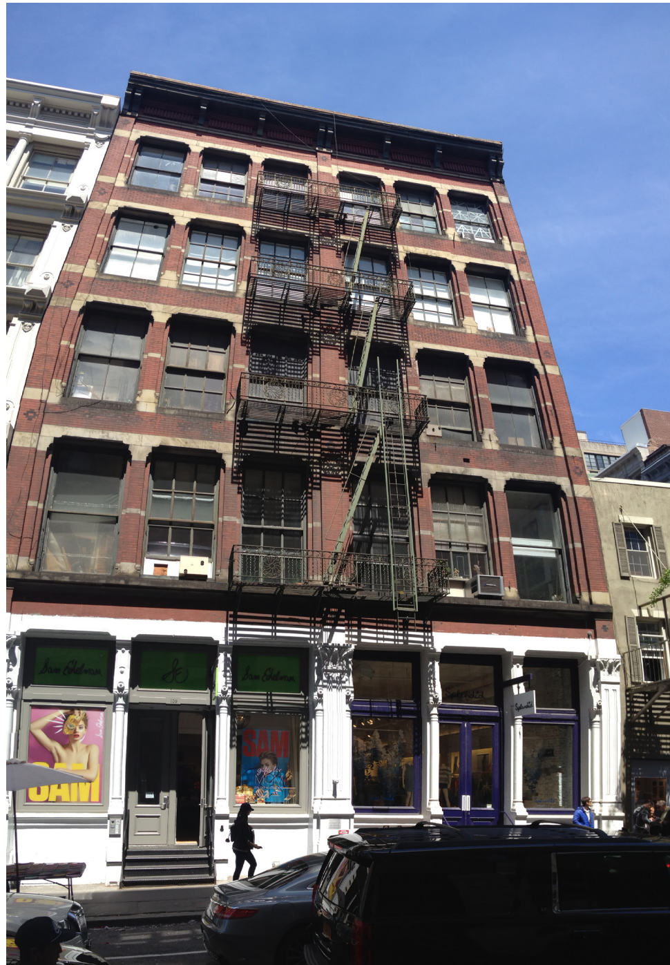
Elevation of full building facade from Spring St. (North side)
