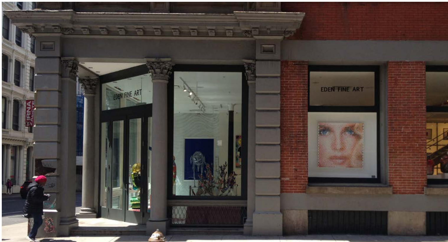
Eden Fine Art, 470 Broome St. (One block south, one block west of proposed work) Bulkhead fill replaced with glazing, historic bulkhead trim maintained
