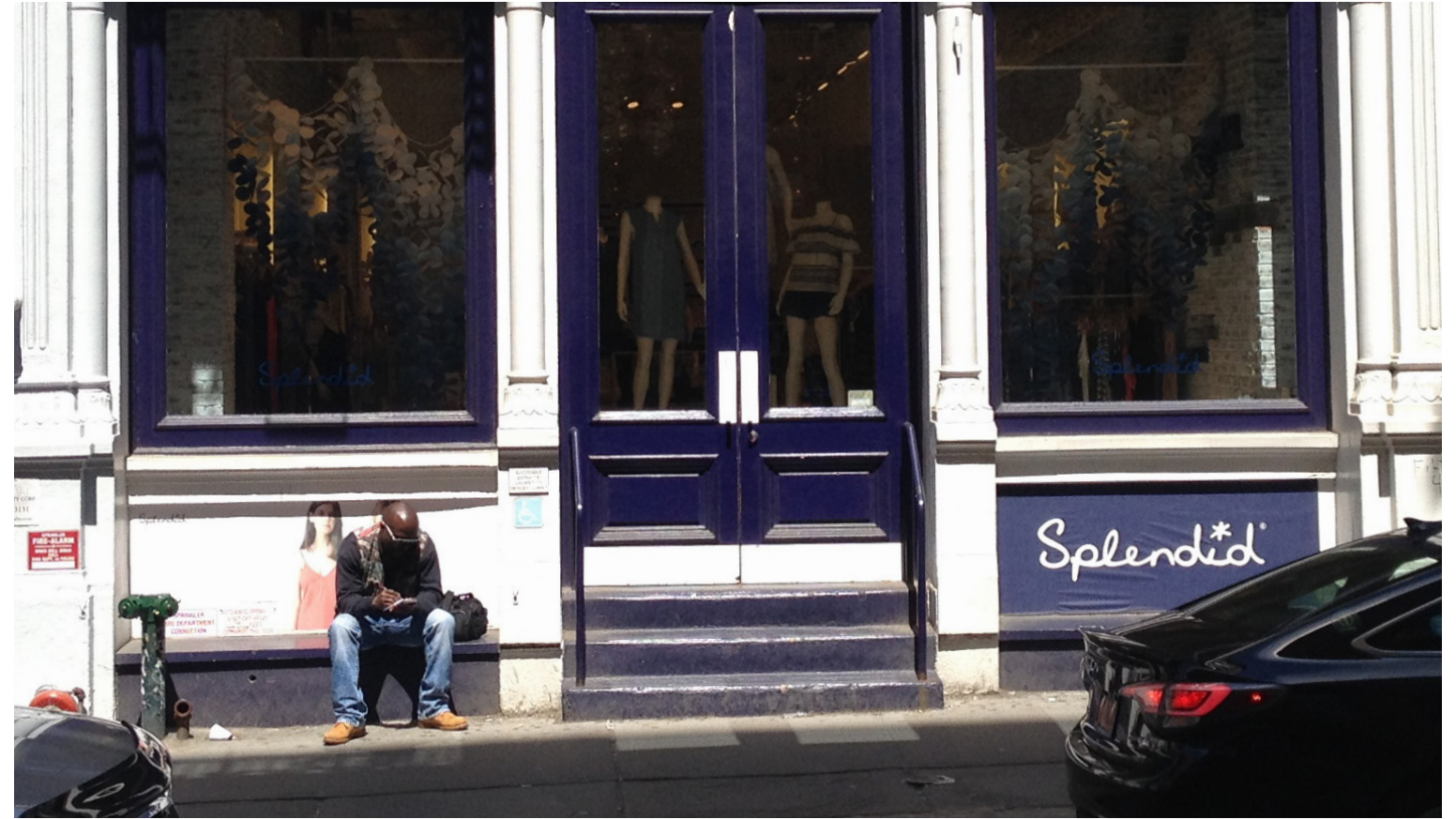
Partial Facade Photo Showing Existing Bulkheads
