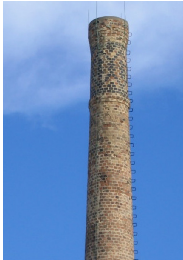
Superior Ink (demolished) 70 Bethune Street
