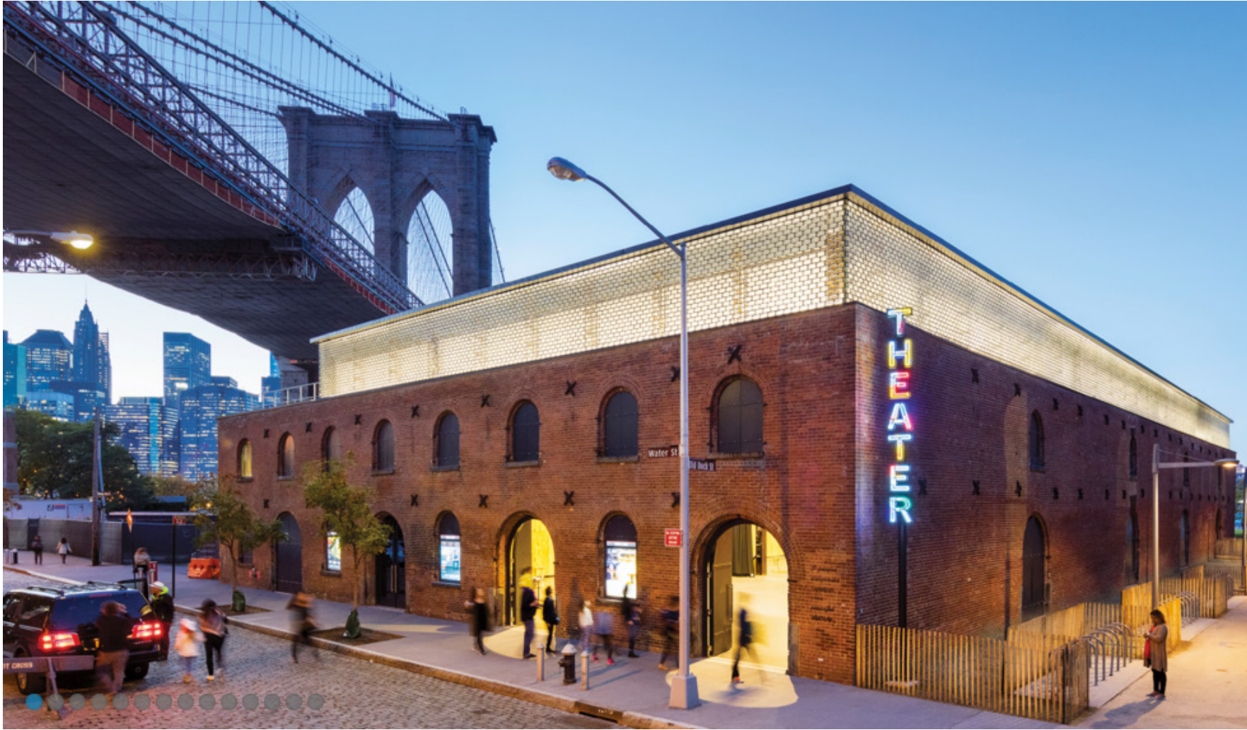
St. Ann's Warehouse, DUMBO
