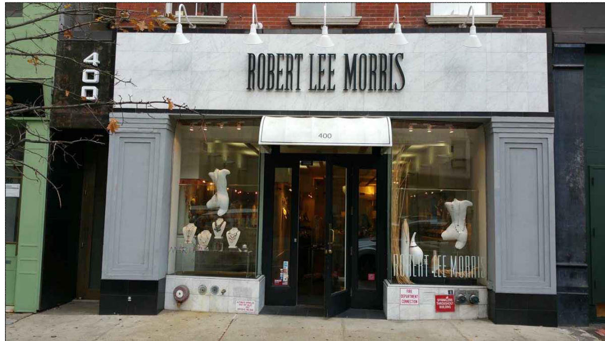
1 PREVIOUS EXTERIOR STOREFRONT PHOTO NTS
