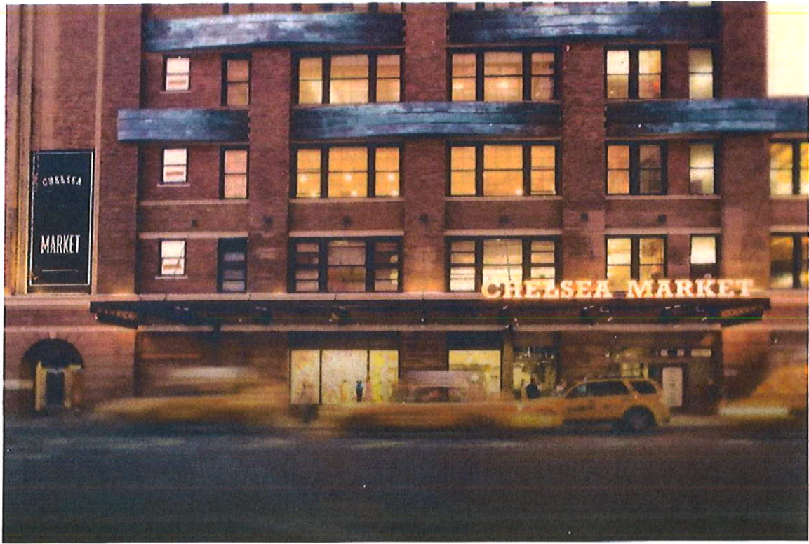
Exterior of building
