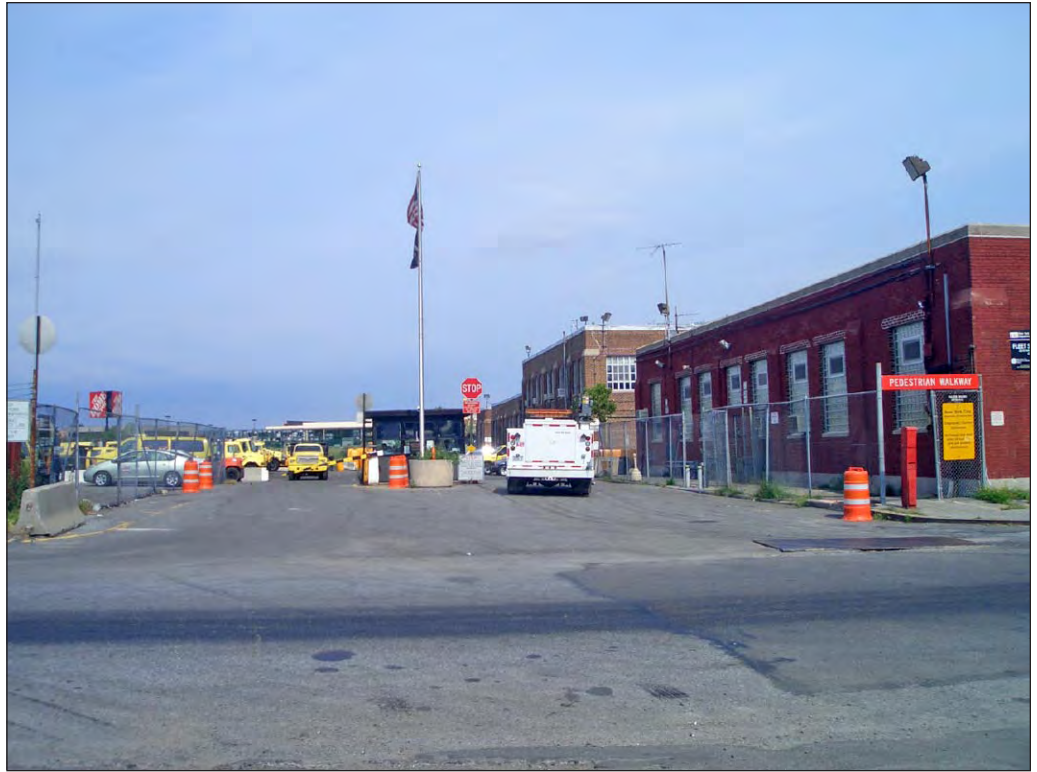
New York City Department of Transportation site 18
