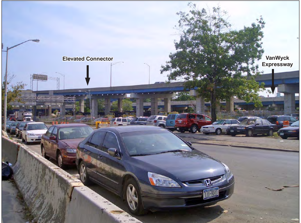
Elevated transportation structures surrounding District 12
