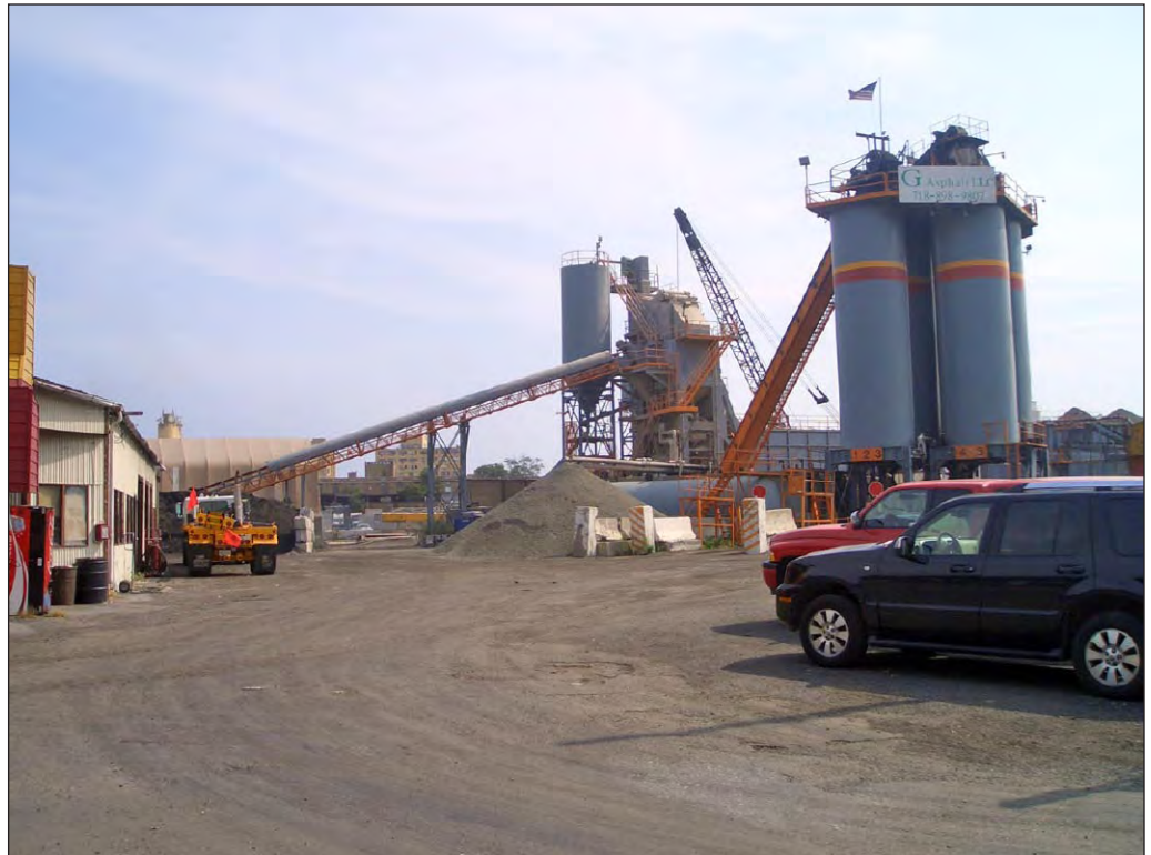
Asphalt plant near Northern Boulevard and VanWyck Expressway 19
