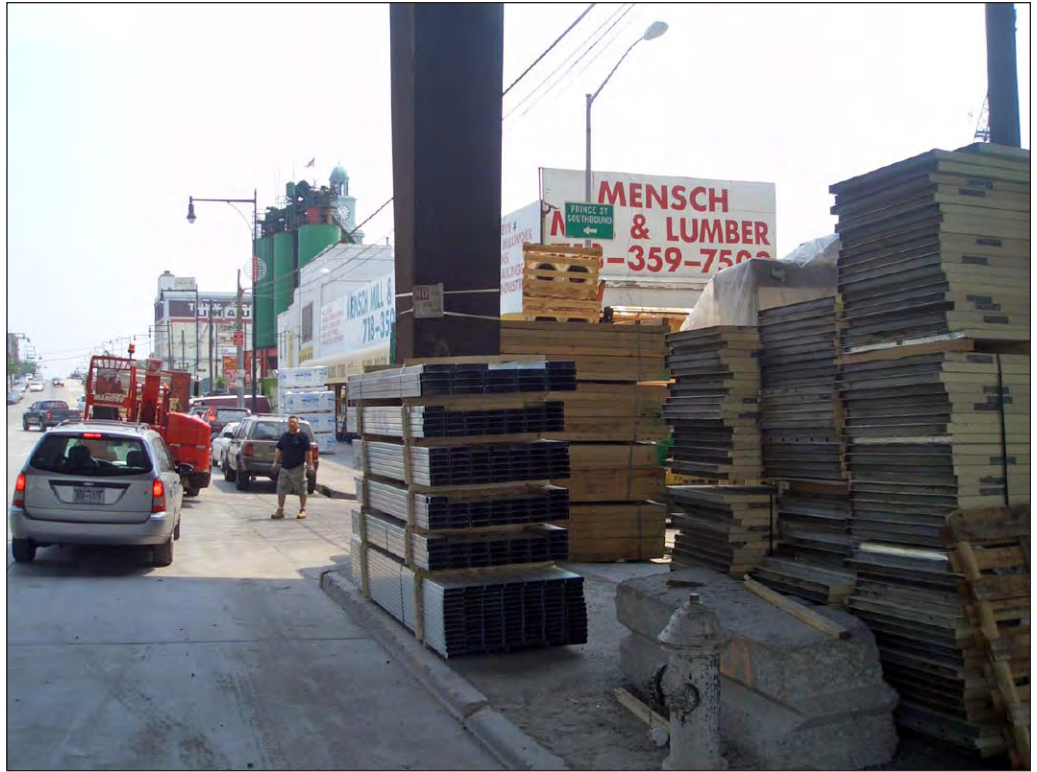
Lumber processing site, view south along College Point Boulevard 24
