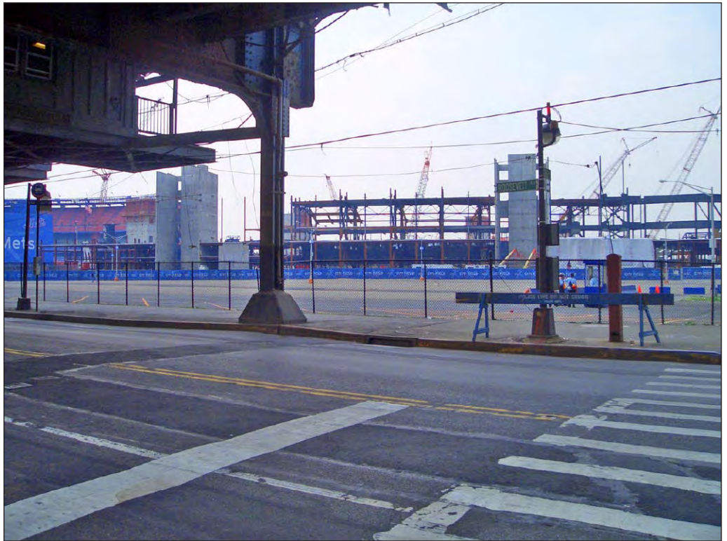
Citi Field Stadium under construction, view north from Roosevelt Avenue 31
