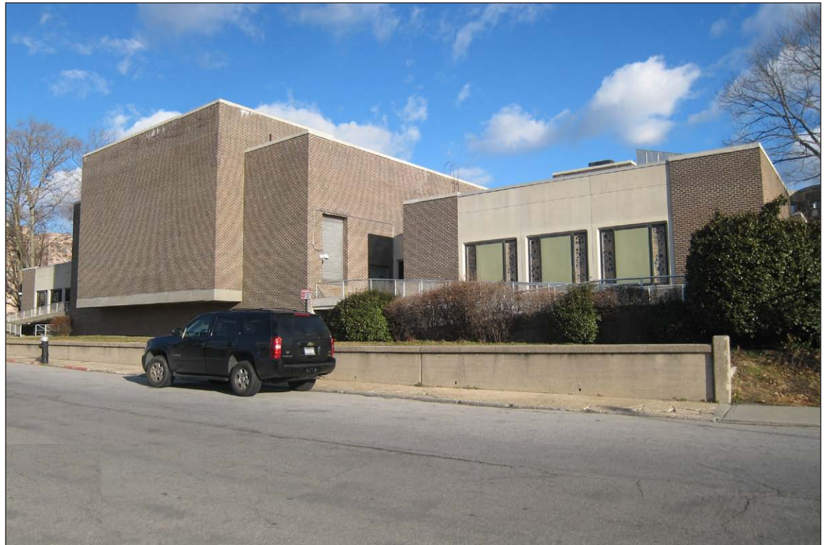
Activities Building/Building J—South facade 7
