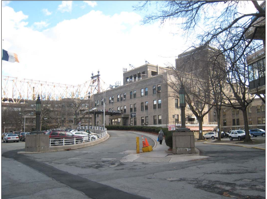
Administration Building/Building E—West facade’s primary entrance and access ramp 1
