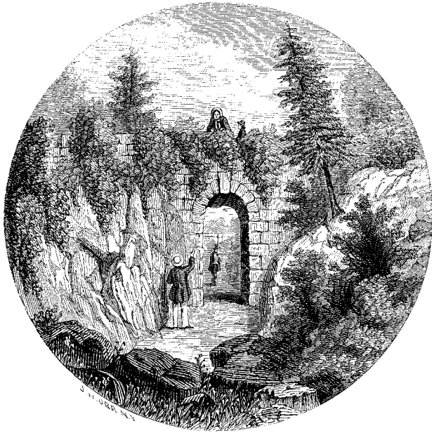
ROUGH STONE ARCHWAY IN THE RAMBLE
