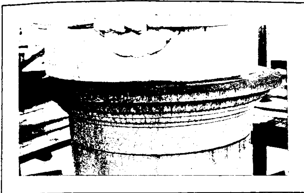
Effects of Vibration and Poor Resetting After Subway Construction
