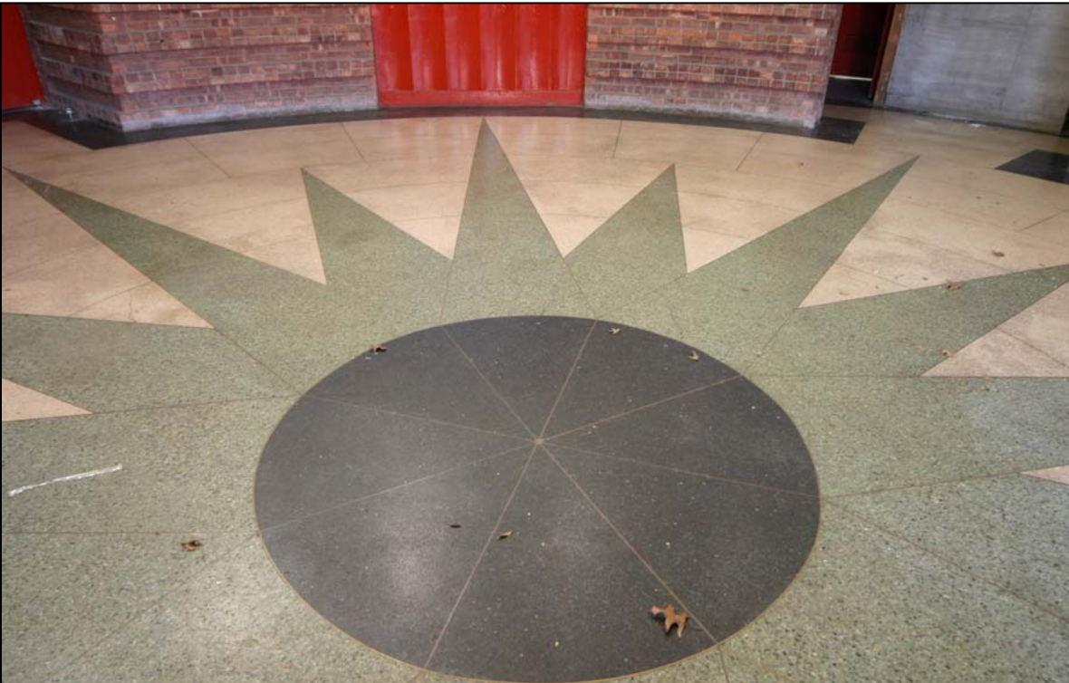
Tompkinsville (Joseph H. Lyons) Pool Bath House Interior: Terrazzo Floor, Lobby Photo: Carl Forster, 2007
