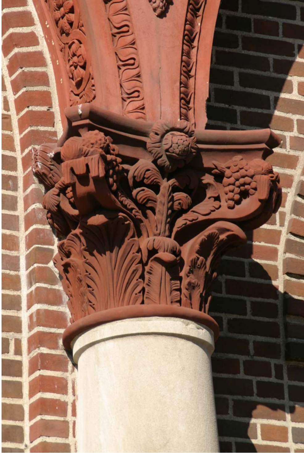
New York Public Library, Hunts Point Branch Detail, terra-cotta capital Photo: Christopher D. Brazee, 2009
