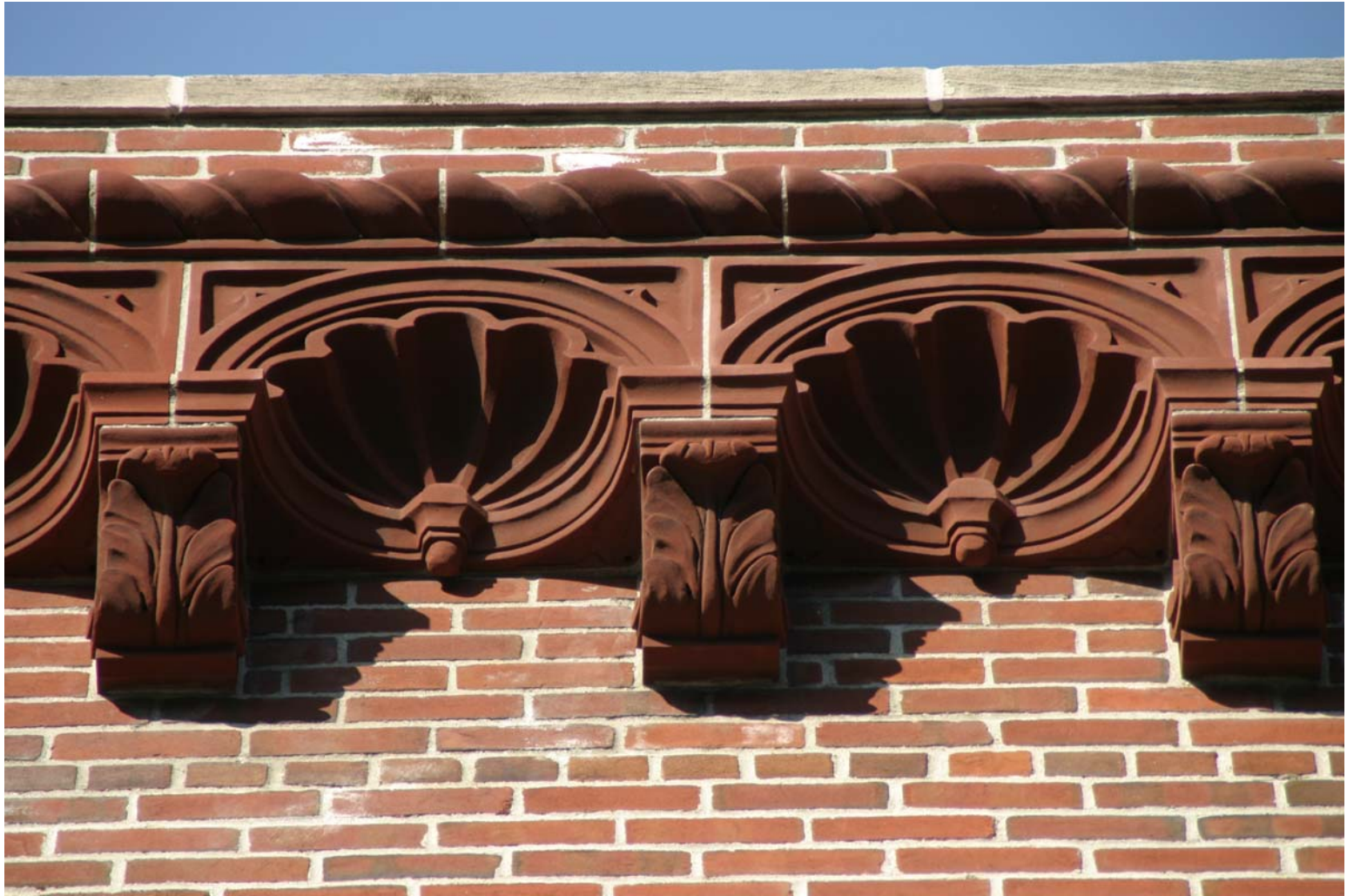
New York Public Library, Hunts Point Branch Detail, acanthus-leaf consoles and scalloped niches in the terra-cotta cornice Photo: Christopher D. Brazee, 2009
