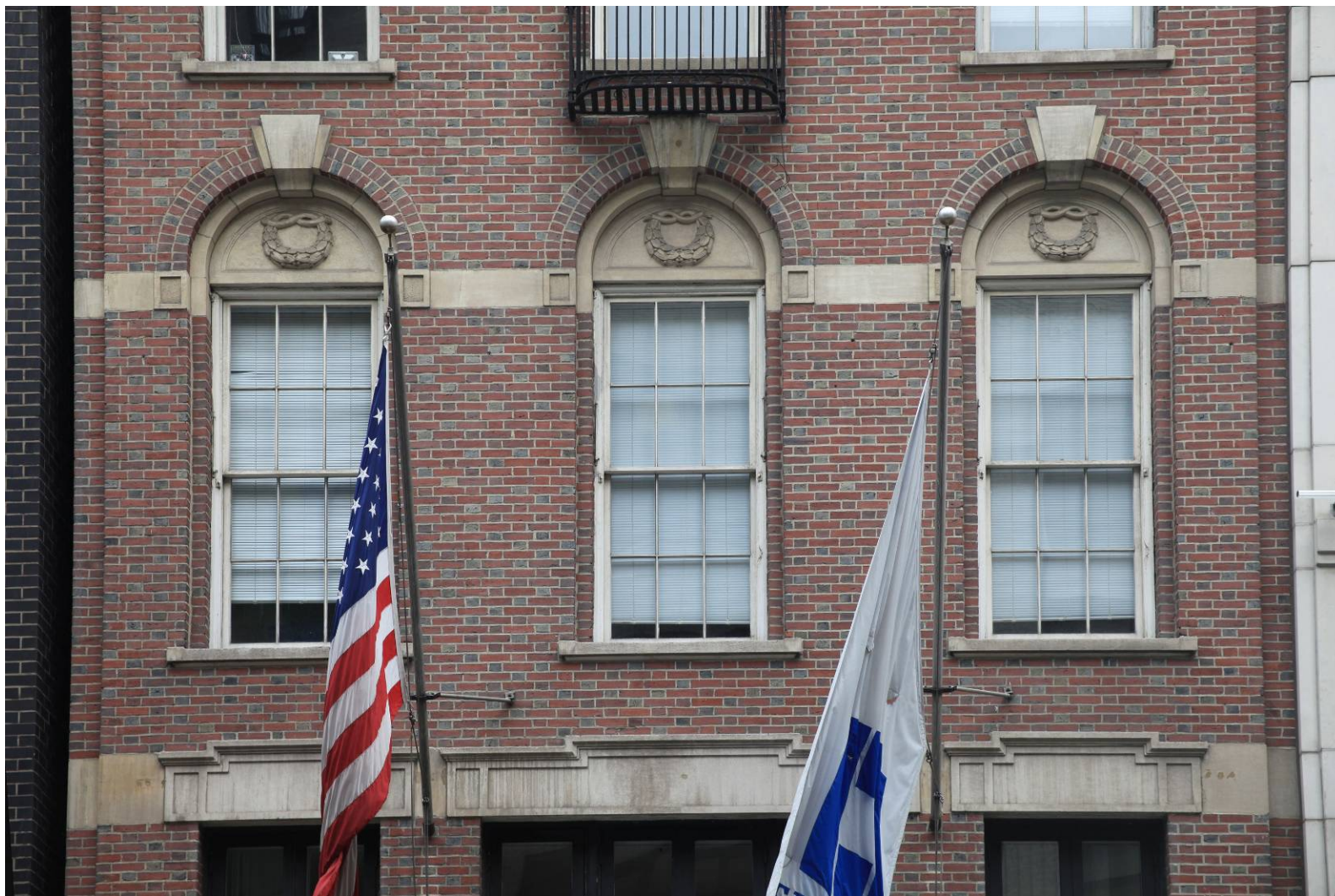
Continuous lintels with Federal-style detailing mark the second and third floors Photo: Christopher D. Brazee, 2009
