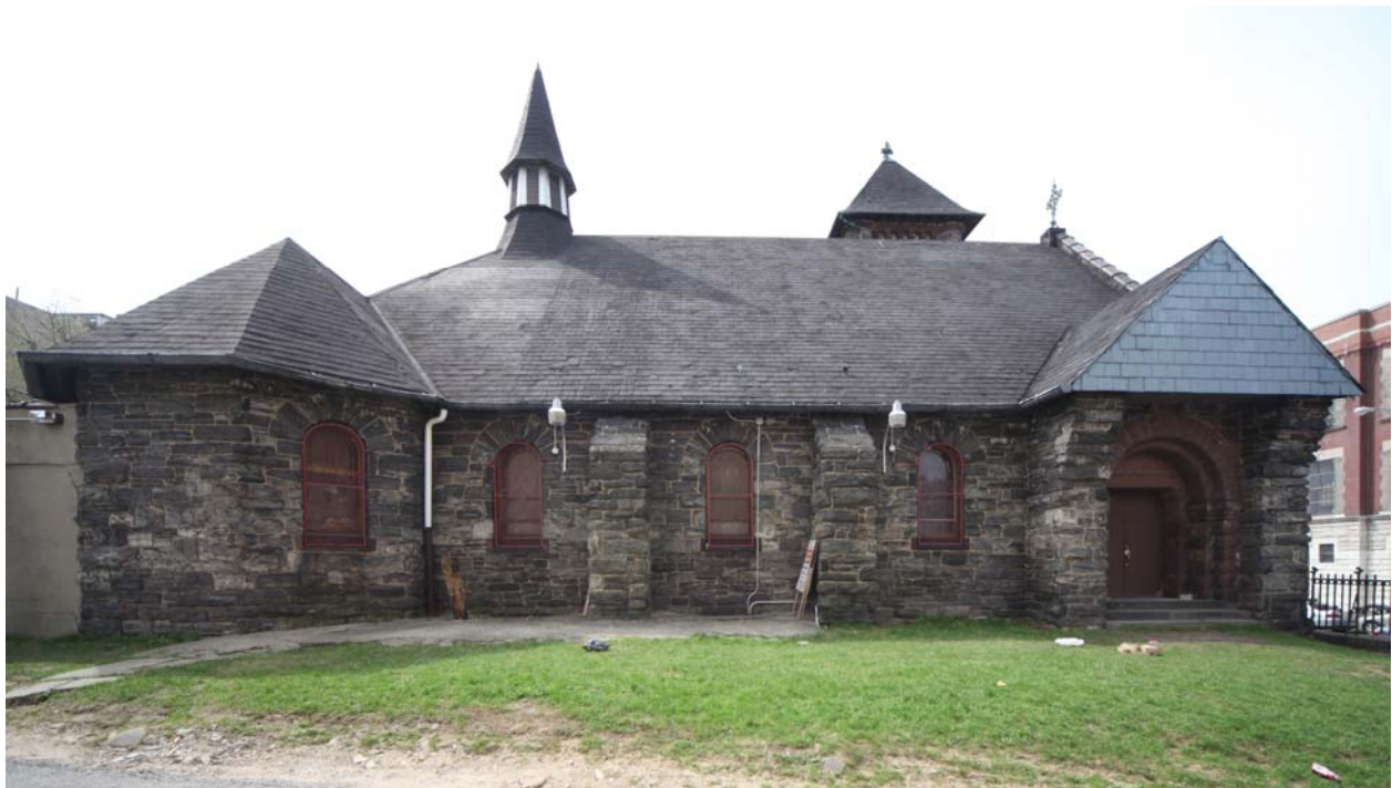
Union Reformed Church of Highbridge (now Highbridge Community Church) North facade
