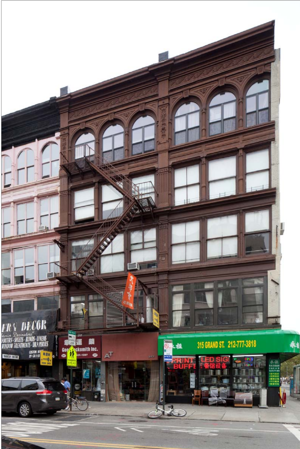
Edward Ridley & Sons Department Store Buildings 315-317 Grand Street, southeast corner of Allen Street Photo: Christopher D. Brazee, 2012
