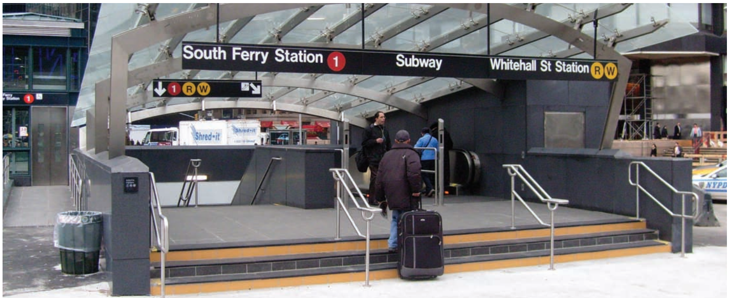
South Ferry subway station (prior to Sandy)
