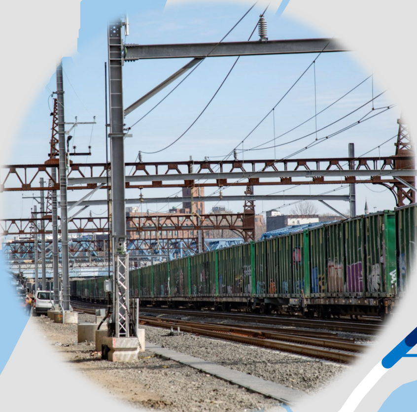
New and old catenary structures at Leggett Interlocking, January 2024
