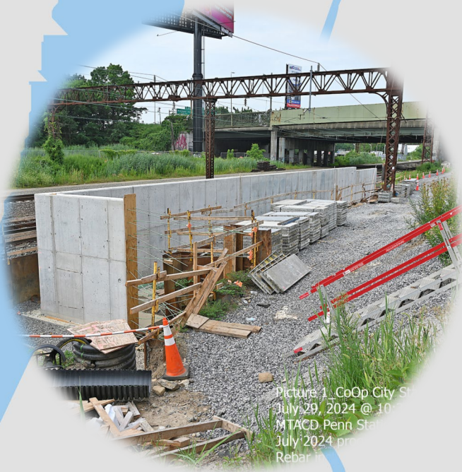
New retaining wall at Co-op City Station site, June 2024
