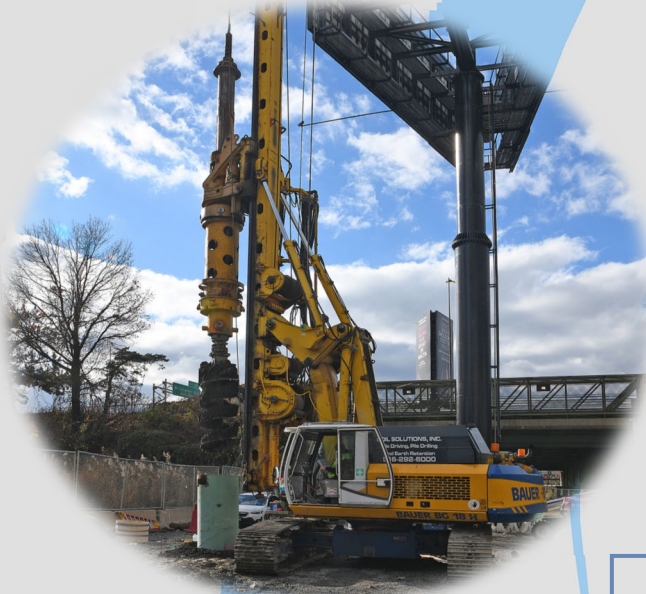
Foundation drilling at Co-op City Substation, November 2023
