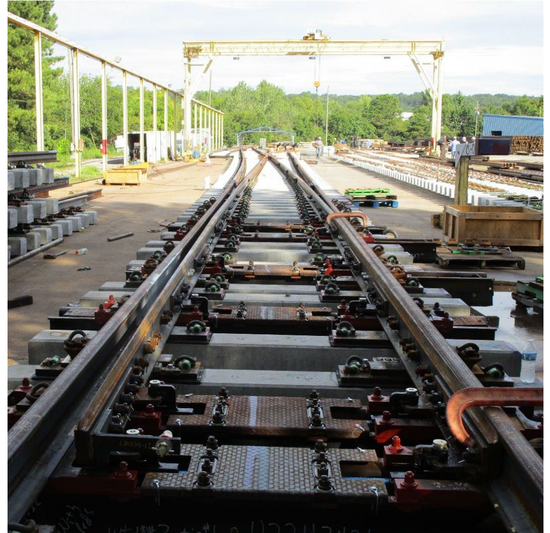
Factory test of fabricated railroad crossovers and switches at Voestalpine Railway Systems Nortrak facility in Birmingham, Alabama, August 2022
