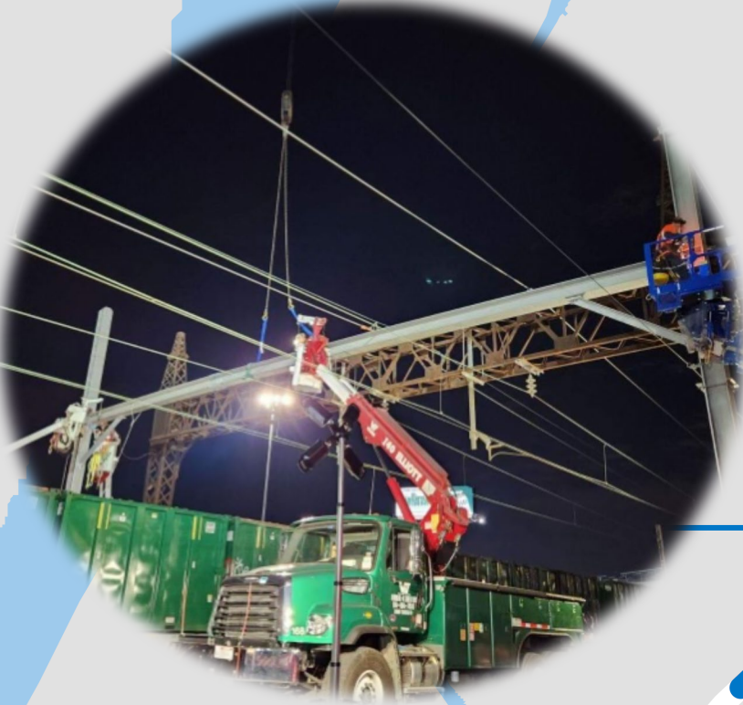
OCS portal installation near Leggett Interlocking, October 2023
