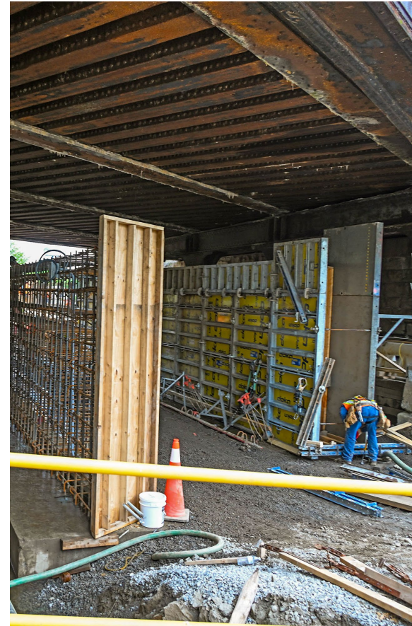
Crews install abutment footings at Pelham Lane Bridge, April 2024
