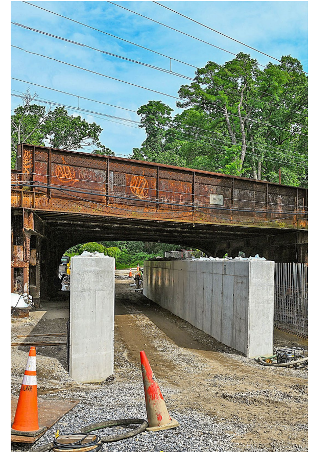
Crews install abutment footings at Pelham Lane Bridge, July 2024
