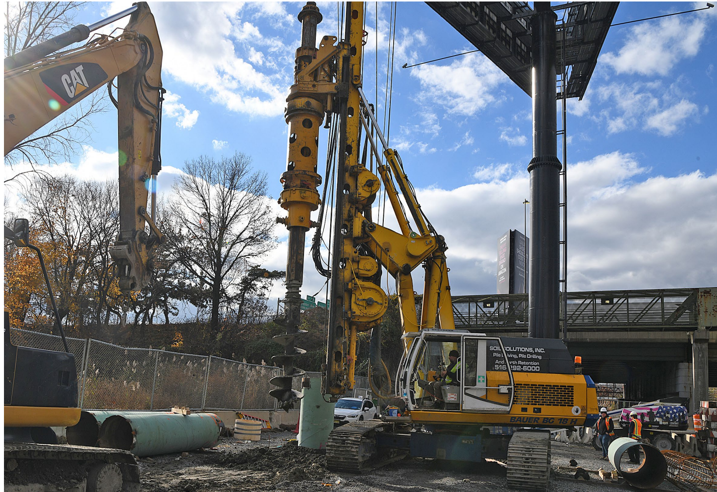
Pile drilling at Co-op City Substation, November 2023
