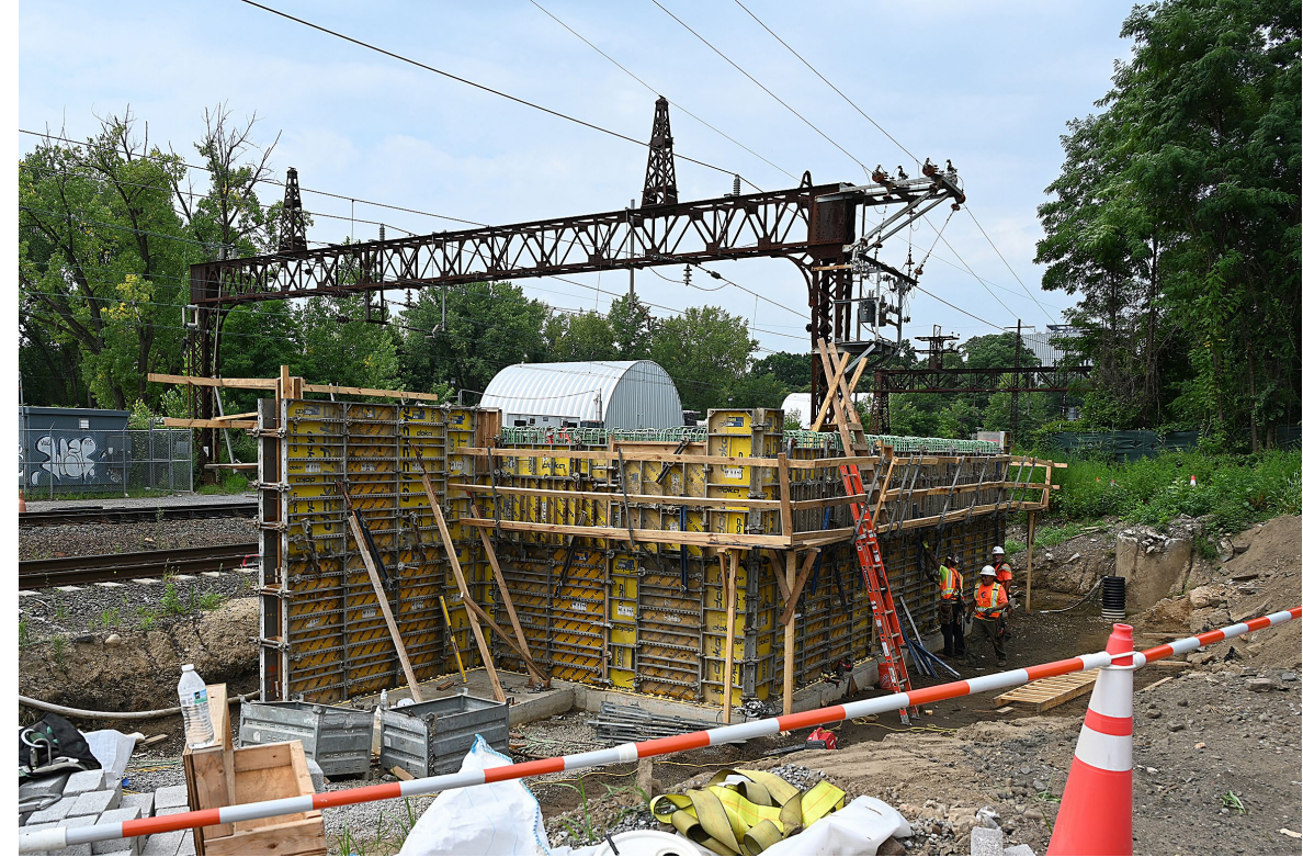
Boiler room formwork at Co-op City Station site, July 2024
