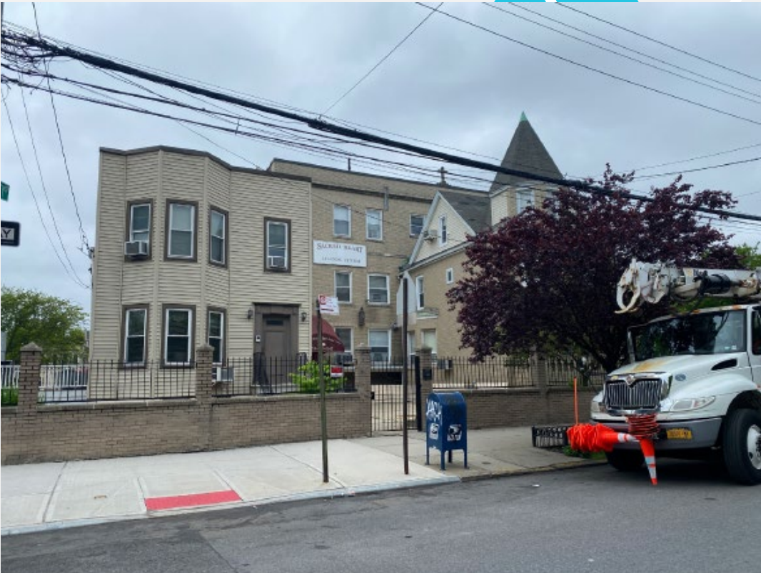
View southwest on Zerega Avenue to the three-story house with a three-story school addition at 1651 Zerega Ave (p/o Lot 78)
