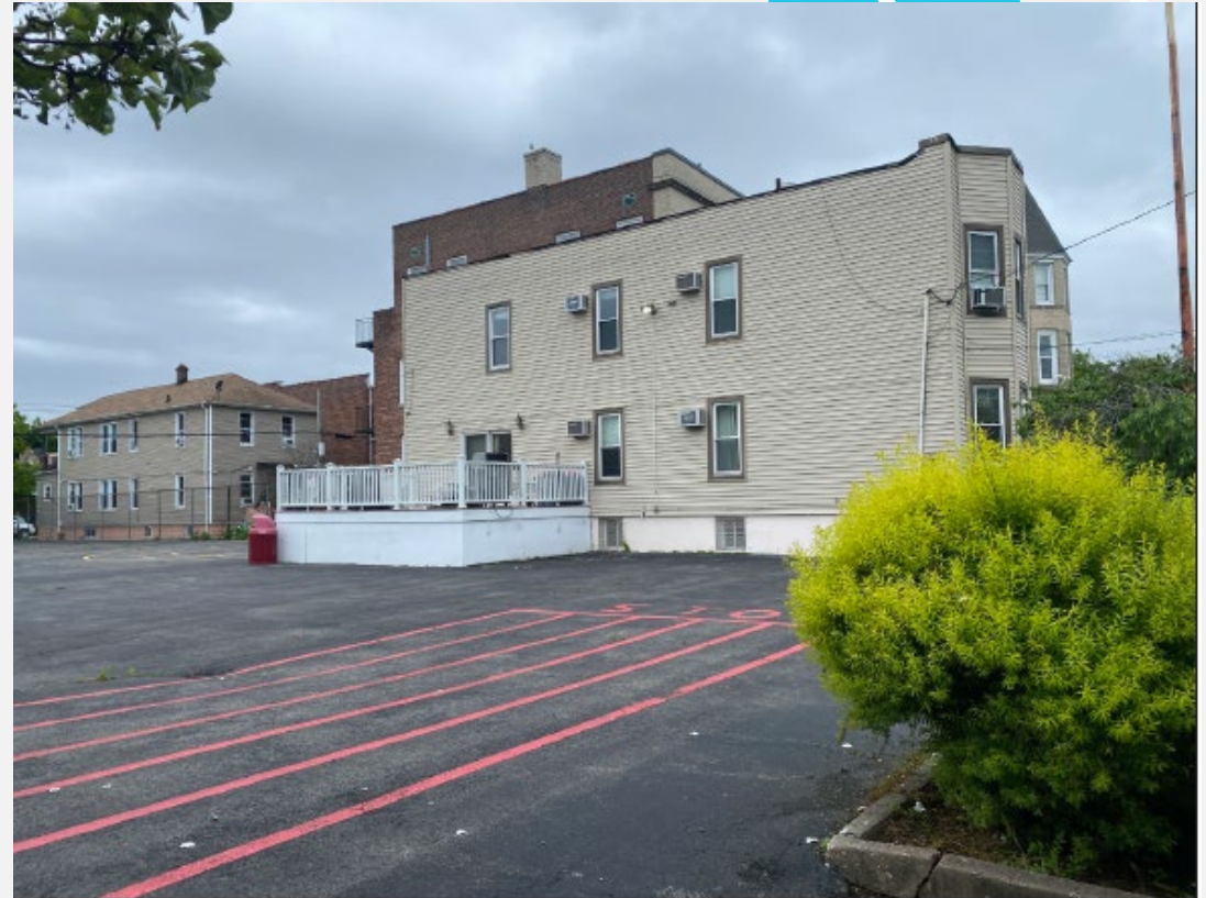
View northwest on Zerega Avenue to the accessory parking lot, including the southeast façade of the two-story house at 1651 Zerega Avenue
