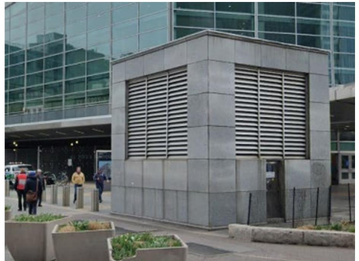
One of four ventilation structures for the Battery Park Underpass
