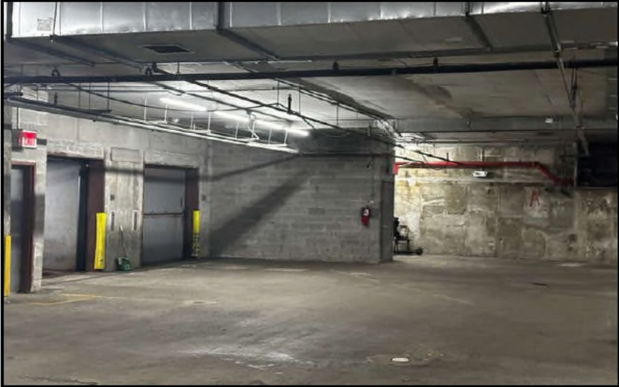
16. Looking northeast at the car elevators in the sub-cellar parking garage.
