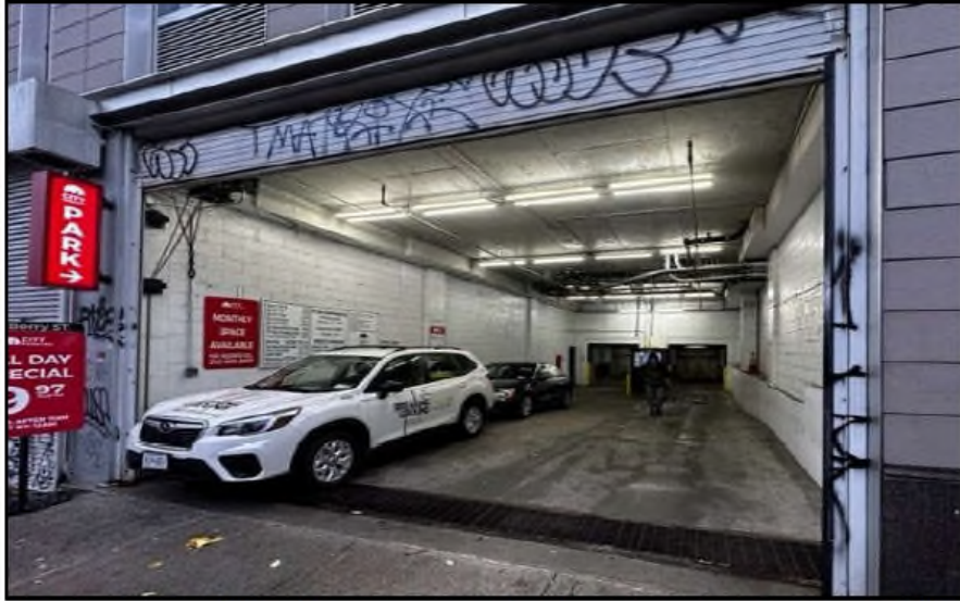
13. Looking east into the entrance of the Development Site's sub-cellar parking garage at the midblock of Berry Street between North 3rd Street and North 4th Street.
