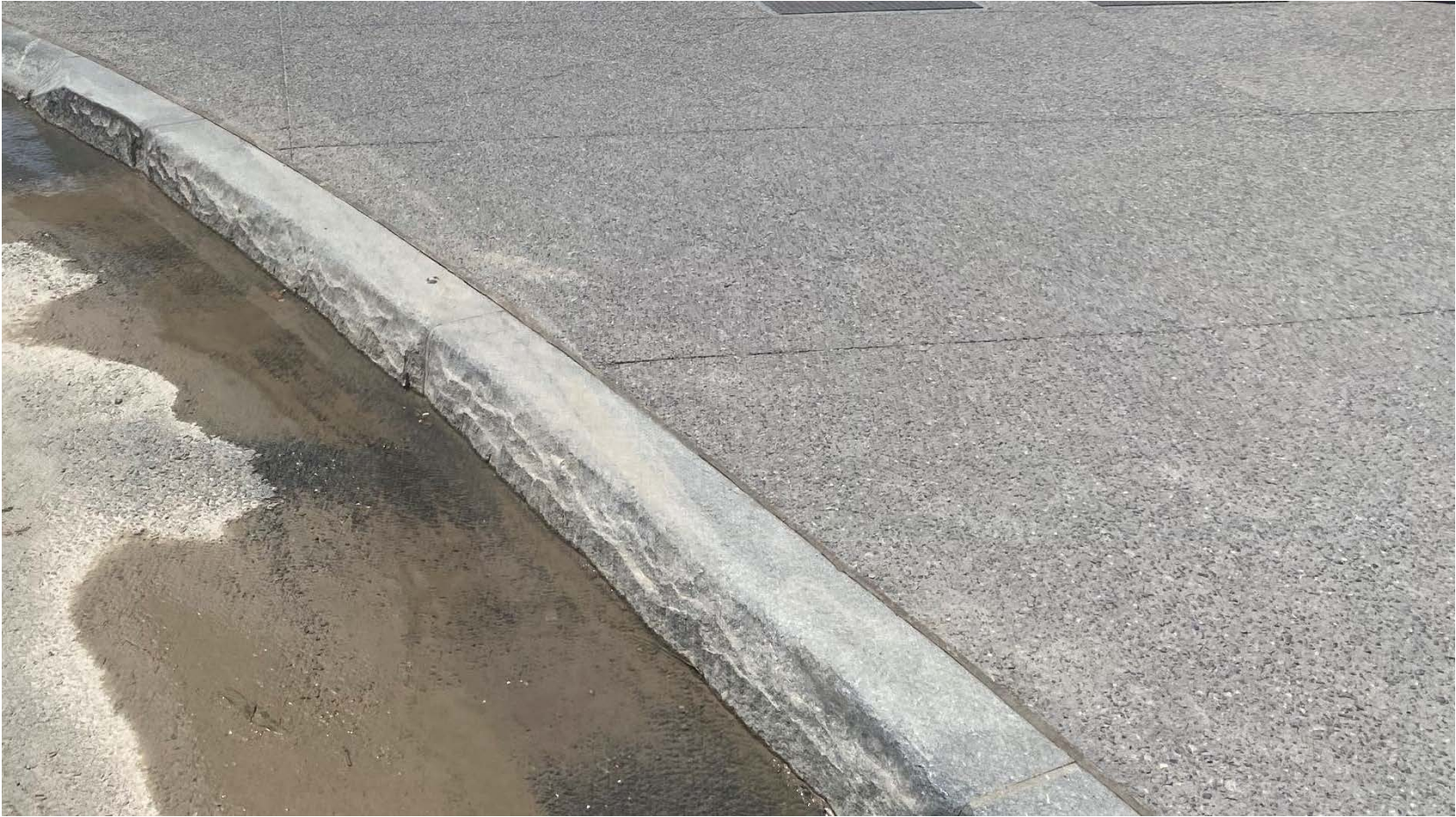
NYCDOT #H-1056 GRANITE CURB NOTE: PHOTO TAKEN AT DOMINO PARK
