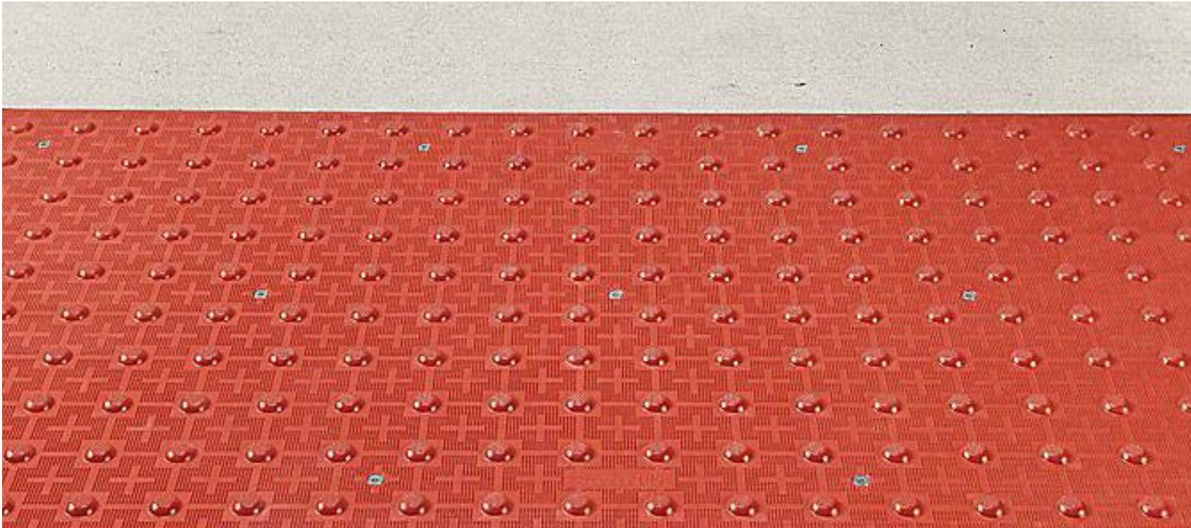
PEDESTRIAN RAMP DETECTABLE WARNING STRIPS
