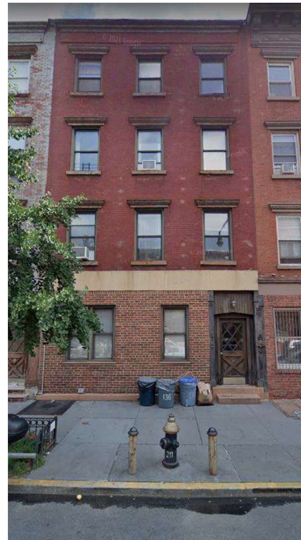
136 Franklin Street ( Existing Condition)
