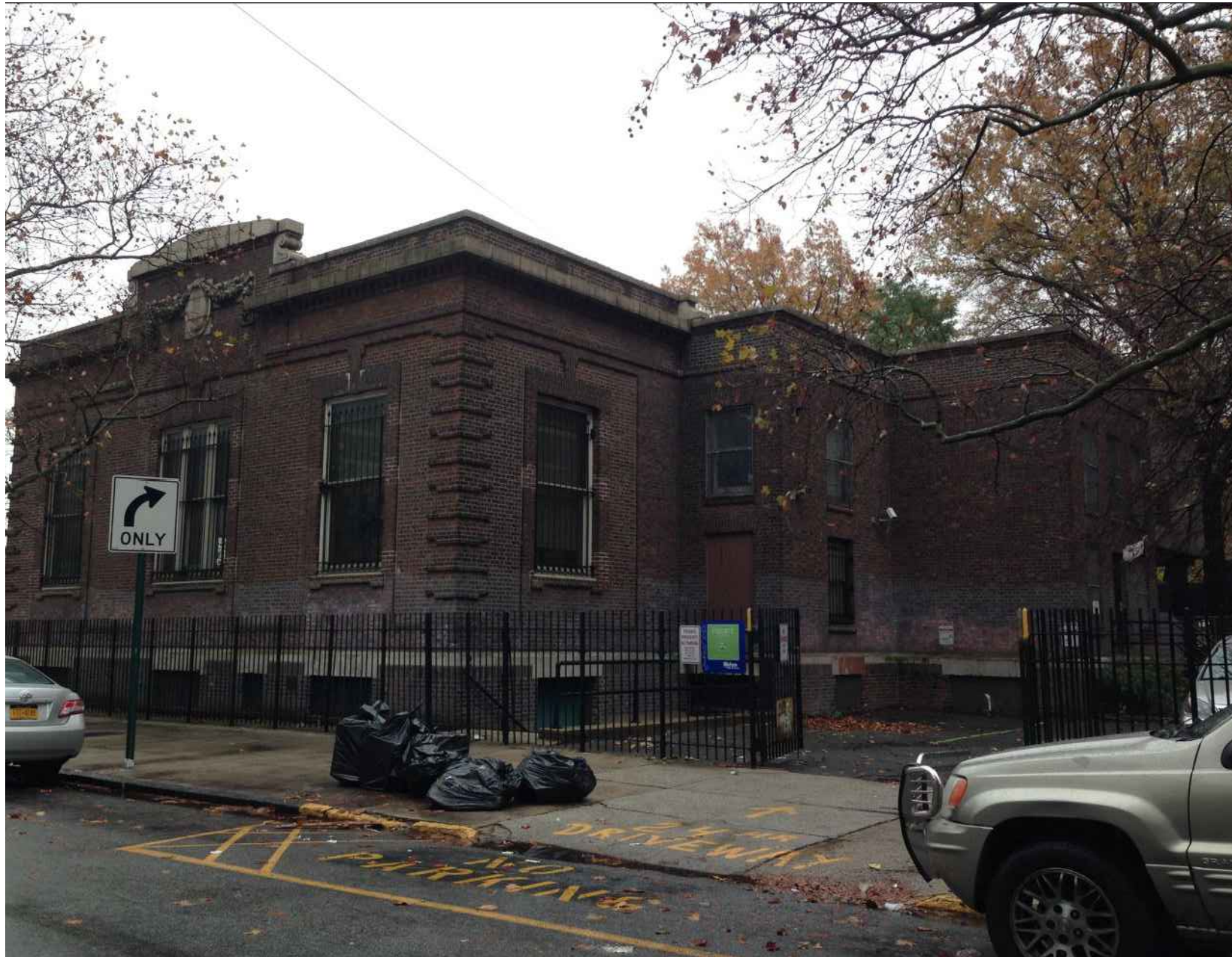
PHOTO 3: VIEW OF NORTHWEST BUILDING FACADE FROM SEIGEL ST
