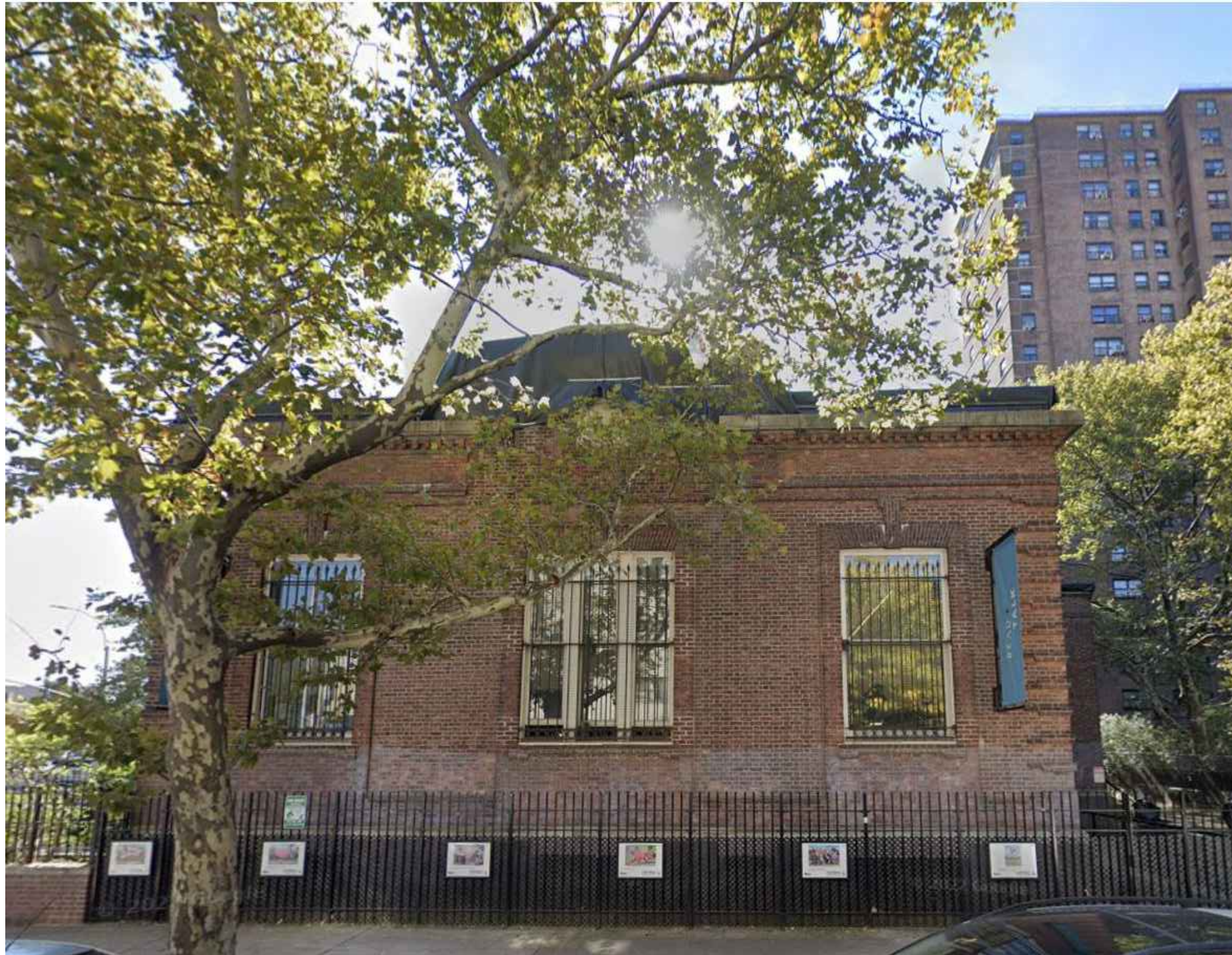
PHOTO 2: VIEW OF NORTH BUILDING FACADE FROM SEIGEL ST
