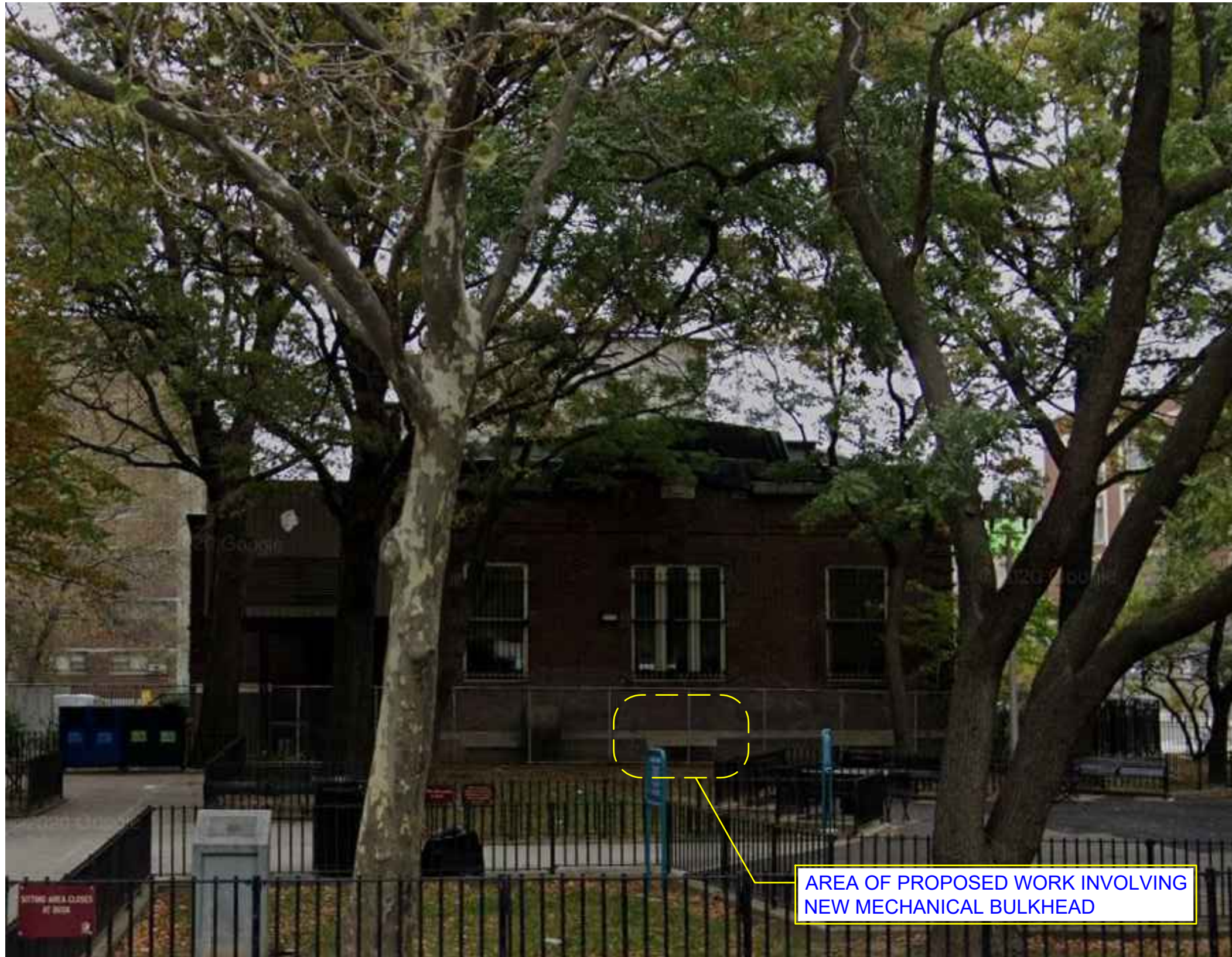
PHOTO 5: VIEW OF SOUTH BUILDING FACADE FROM MOORE ST
