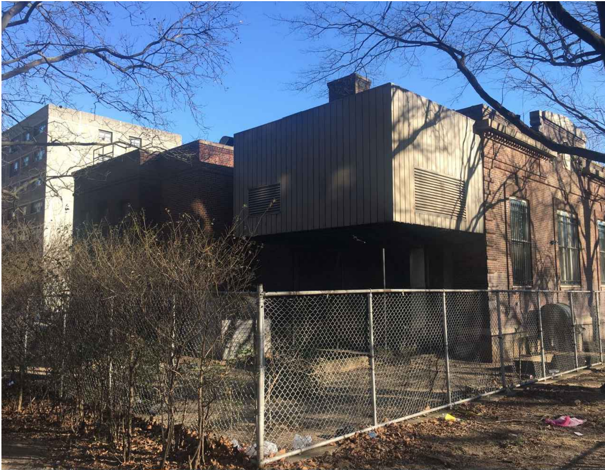
PHOTO 4: VIEW OF SOUTHWEST BUILDING FACADE FROM ADJACENT PROPERTY
