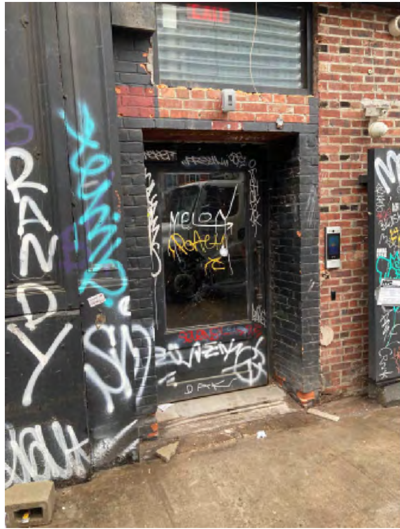
1 PHOTO OF EXISTING DOOR A-102
