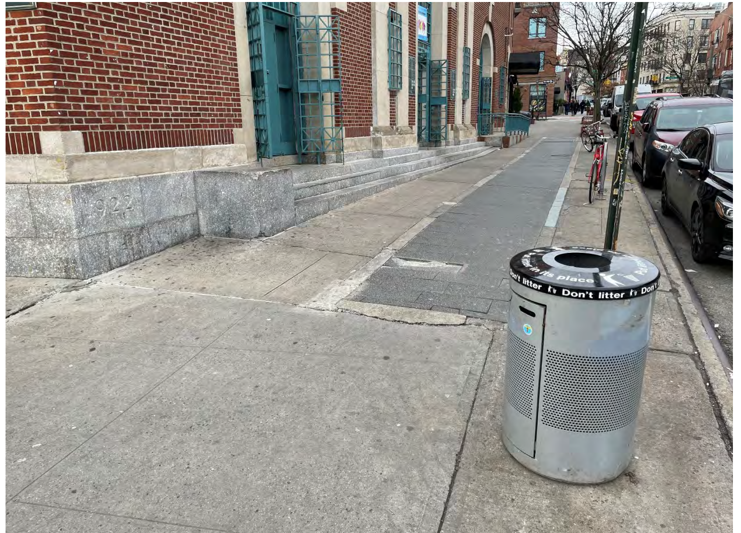
2 – View of sidewalk looking south
