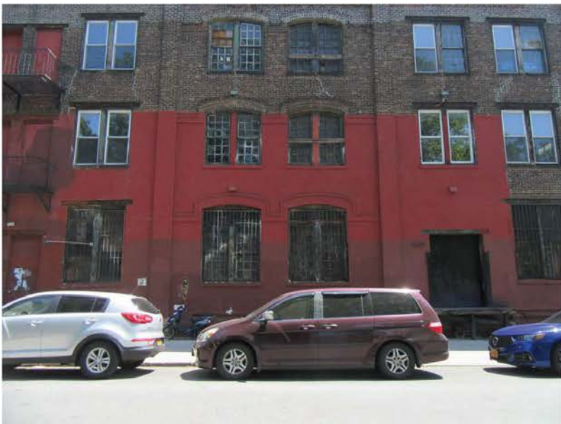
3. View of the Development Site facing northeast from Lorimer Street.
