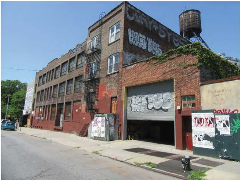
12. View of the Development Site facing west from Driggs Avenue.
