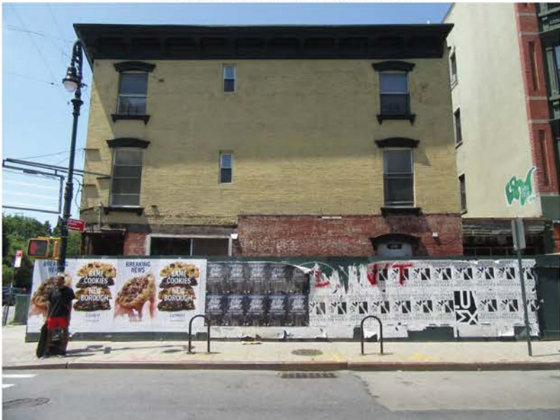
18. View of the Project Area facing southwest from Manhattan Avenue.
