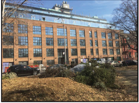
4 LORIMER AVE - VIEW EAST
