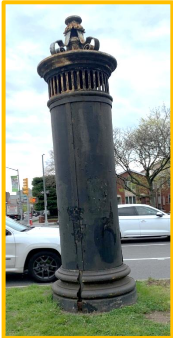
Restore Ornamental Cast Iron Air Intake Stack
