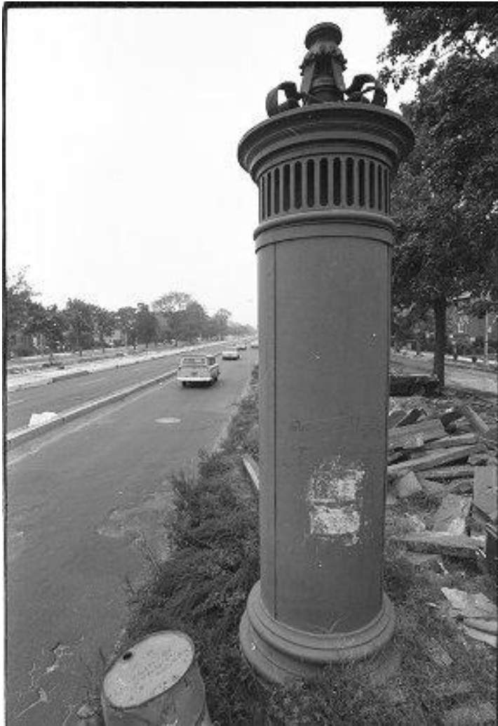
Ornamental Cast Iron Air Intake Stack (1974)
