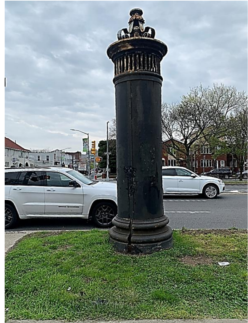
Photo 2 – Original Dry Well Air Intake Stack
