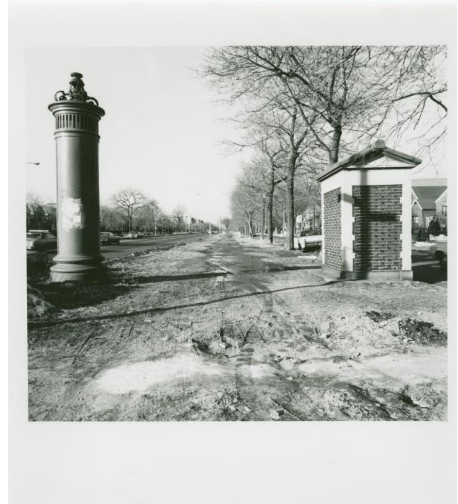
Ornamental Cast Iron Air Intake Stack (1978)
