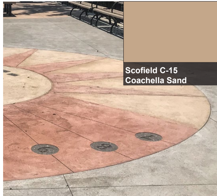
Saw Cut Integral Colored Concrete Pavement
