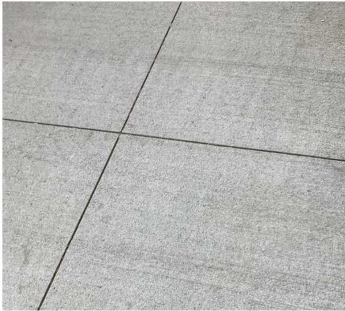
Saw Cut Standard Concrete Pavement Cut
