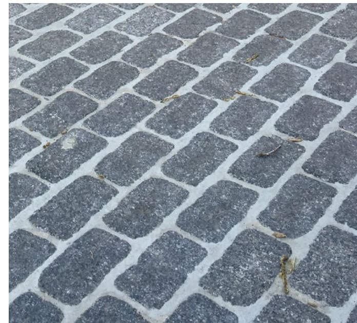
Reset Granite Block with Mortar Joints
