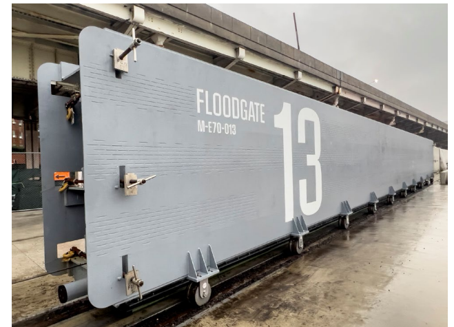
Storm Surge Gates
