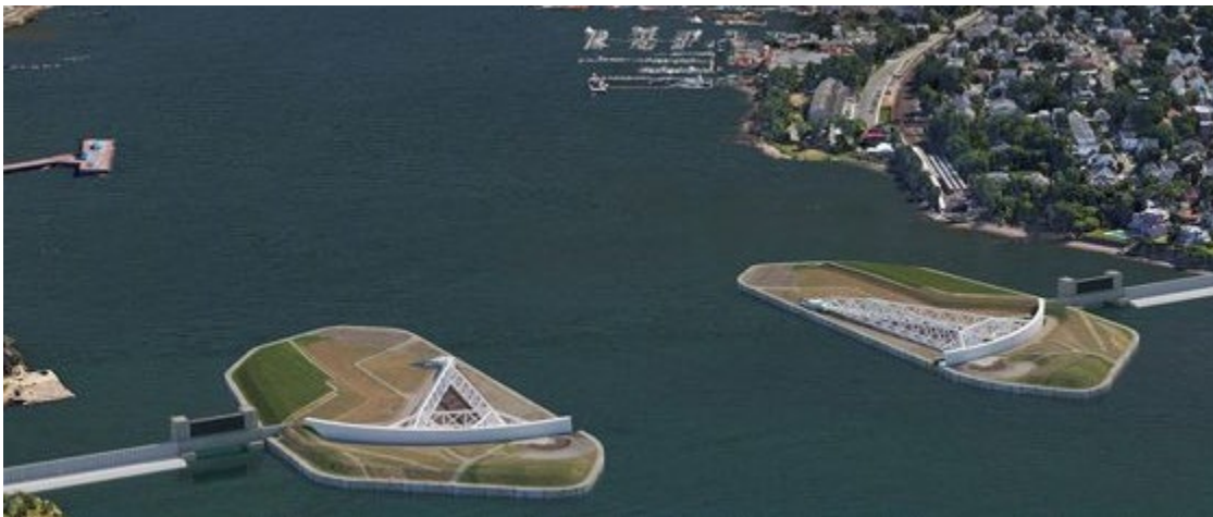
Sea Walls and Sea Gates
