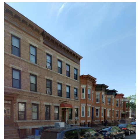
Moffat Street between Wilson and Central avenues
