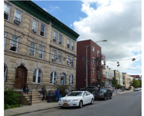
Midblock: Troutman Street between Evergreen and Bushwick avenues
