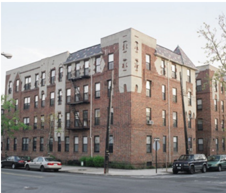
Stockholm Manor has been acquired, refinanced, and will soon be rehabilitated to meet Passive House design standards.
