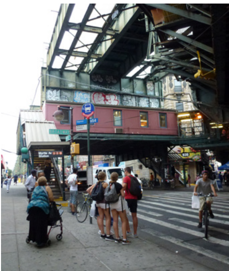
Myrtle Ave Station on the J, Z, M subway lines
