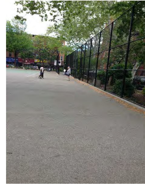
Full Depth Asphalt
