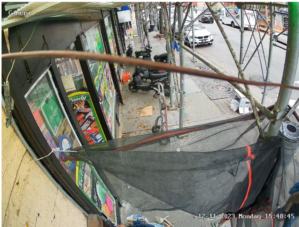
Image #32: D18 Camera Worker with tools (2023-12-11, 172 W. Burnside Ave. Security Camera)
