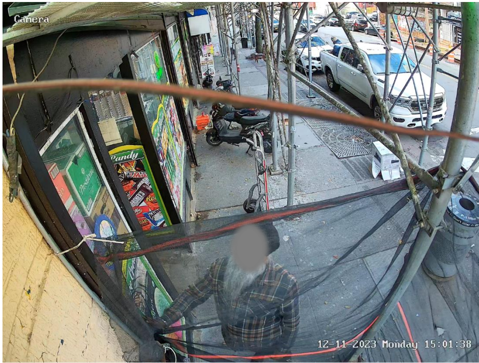
Image #27: D18 Camera Permit Holder inspecting load-bearing masonry pier (2023-12-11, 172 W. Burnside Ave. Security Camera)
