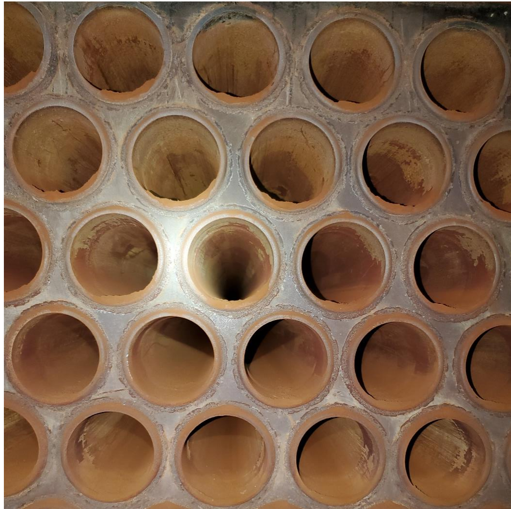
Visual inspection of boiler firetubes
