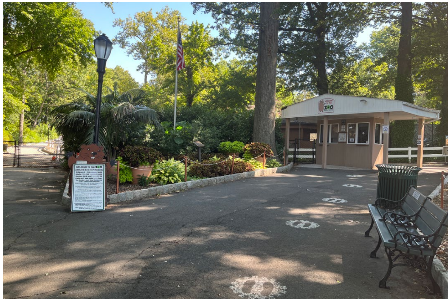
1 Service Access (left) and Ticketing Kiosk (right) See corresponding proposed view on p.17
