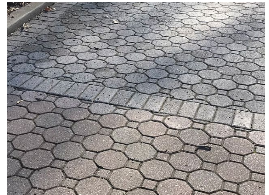
Image of existing pavers
