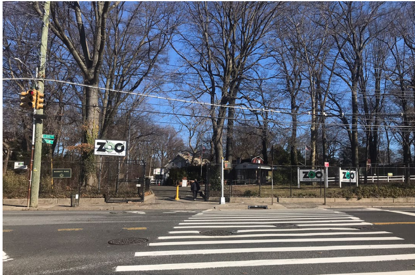
1 Clove Road Entrance showing existing vehicular and pedestrian curb cuts and crosswalk
