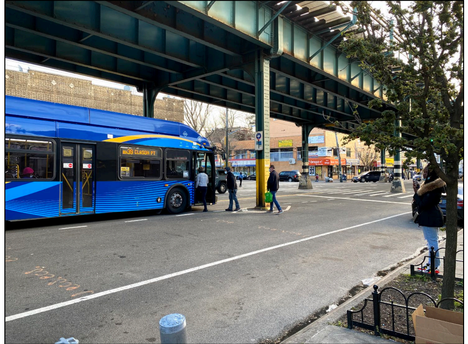
White Plains Road before, inaccessible bus stop required riders to board in the roadway
