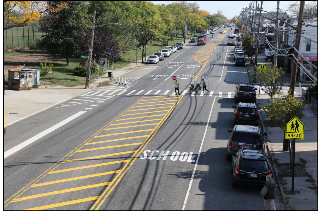
Gerritsen Ave is a 60' wide road that had wide center medians, infrequent signals, and high rates of speeding
