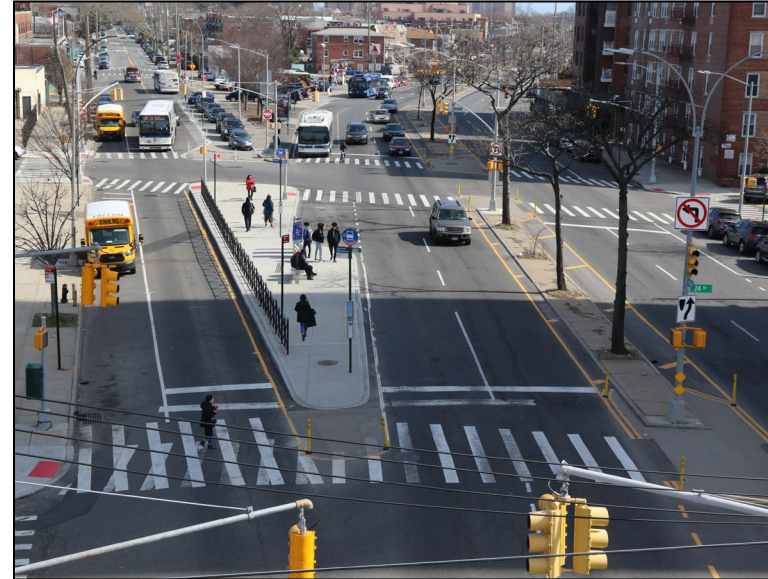
Vision Zero SIP installed on Cropsey Ave installed a bus boarding island, pedestrian space, turn bans, and markings upgrades
