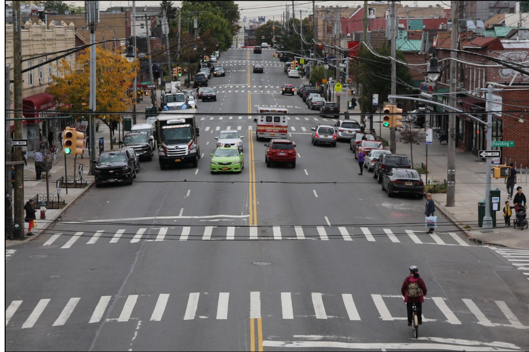
Morris Park Ave is a 60' wide roadway that had two travel lanes and parking in each direction
