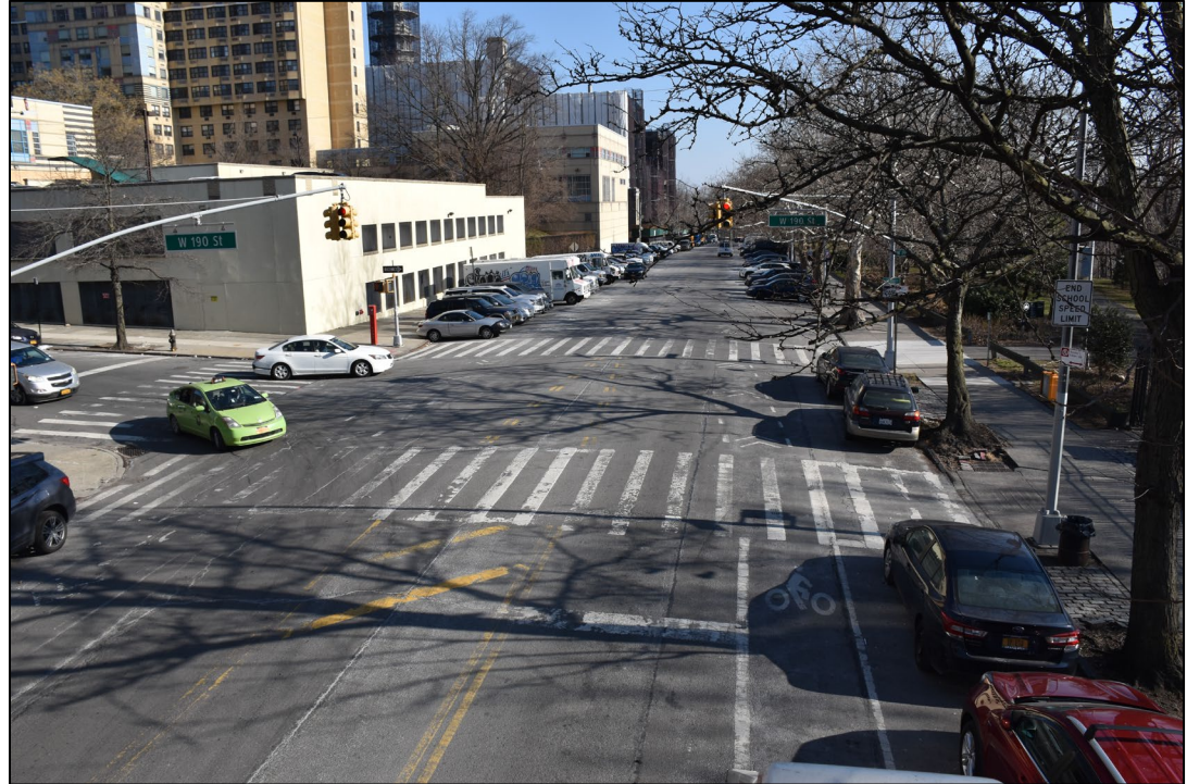
Amsterdam Ave, before. Wide roadway with faded markings encouraged speeding near numerous schools
