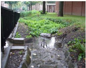
These below-grade landscape features can be installed to catch surface runoff from driveways, sidewalks, and rooftops to prevent excess water from entering the stormwater/sewer system.
