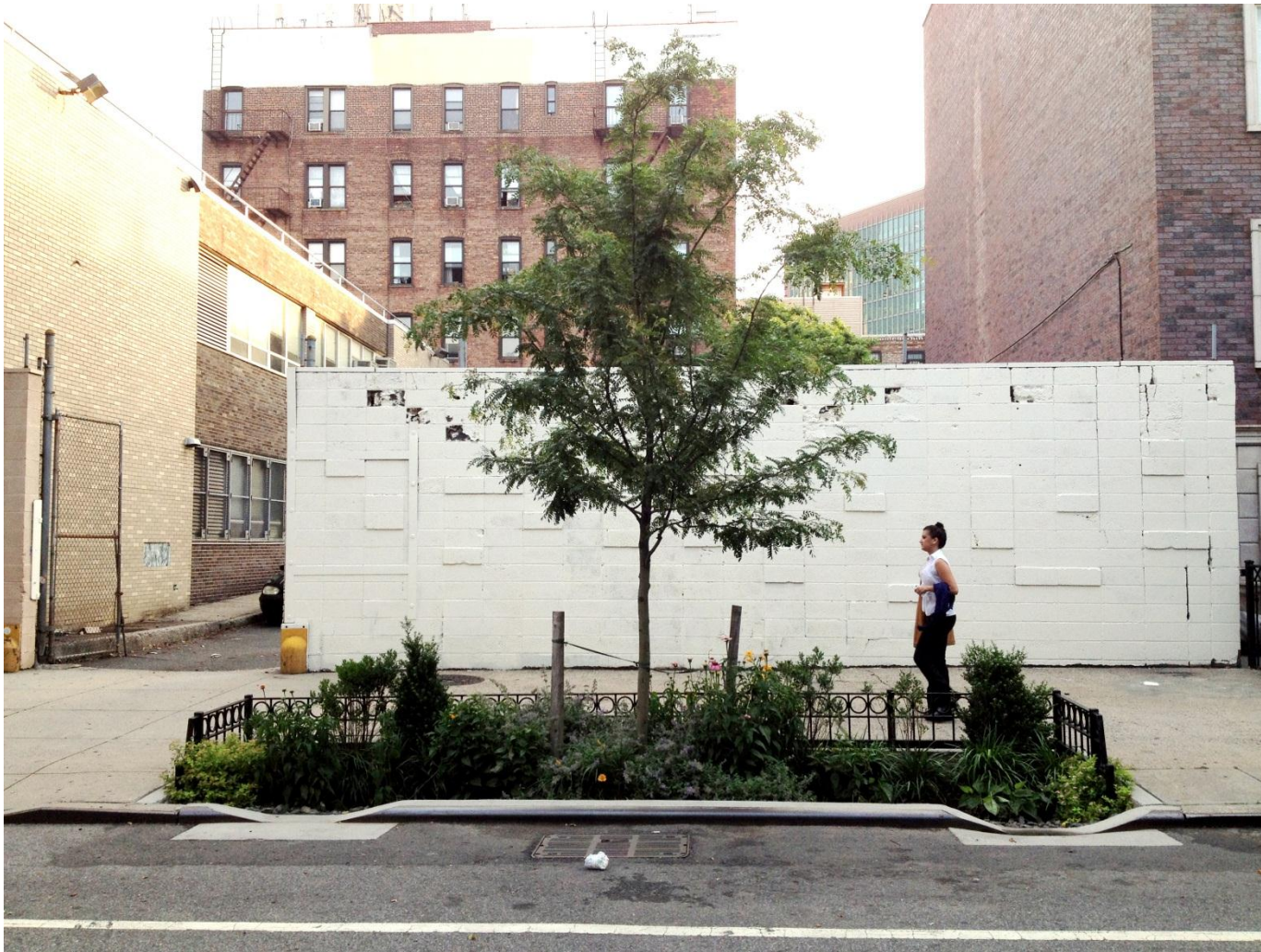
Construction of a ROW Bioswale
