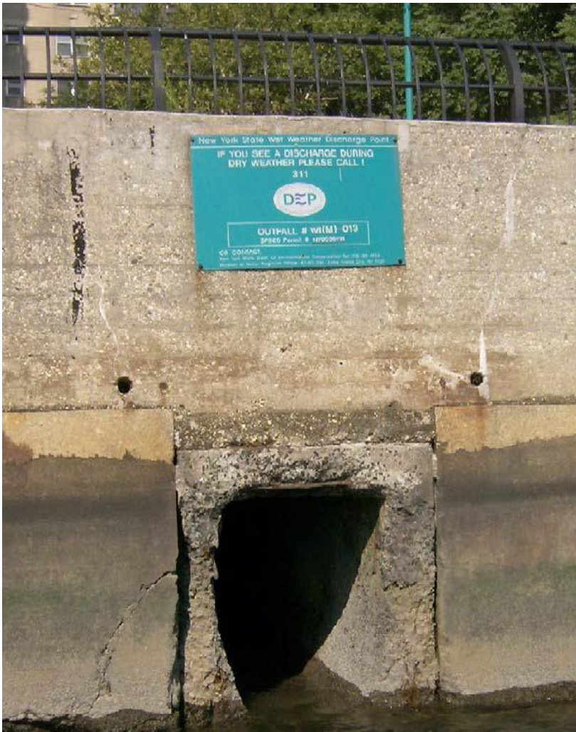
Combined Sewer Outfall
