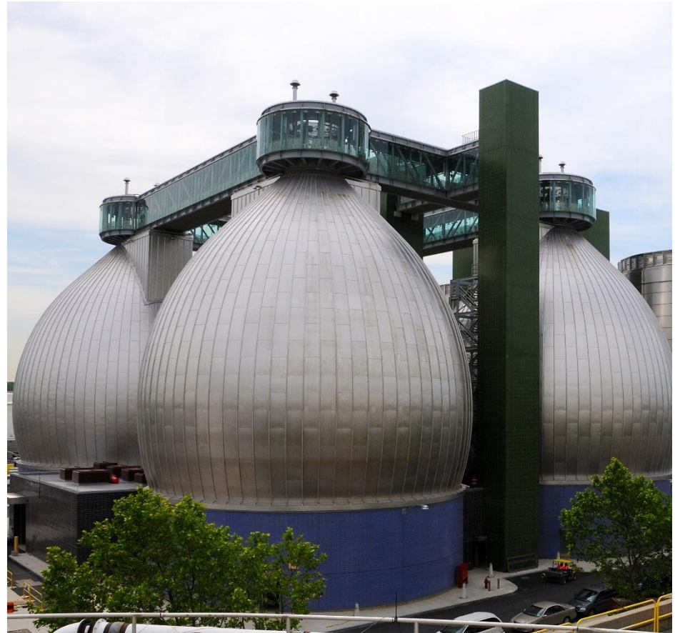
View of the digester eggs at the Newtown Creek Wastewater Treatment Plant
