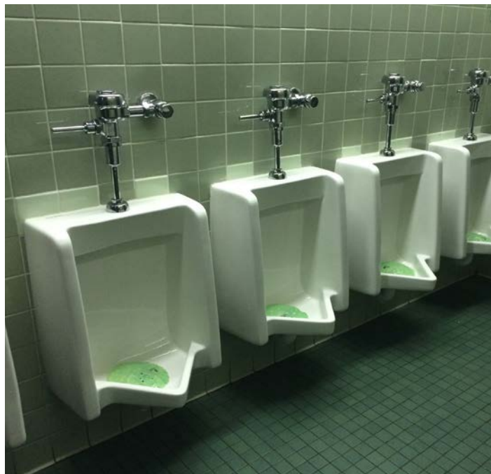
Figure 5: Retrofitted urinals at P.S. 1 in Staten Island
