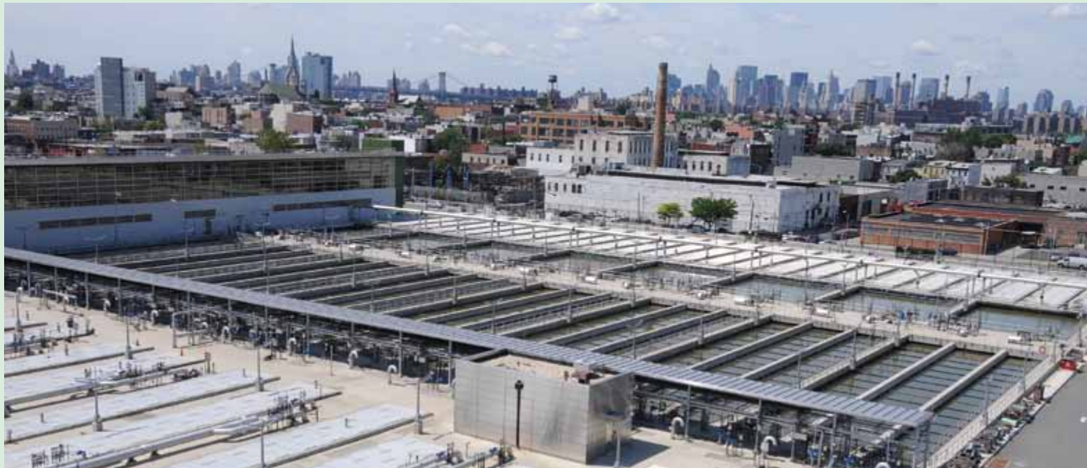
Newly upgraded Newtown Creek Wastewater Treatment Plant
