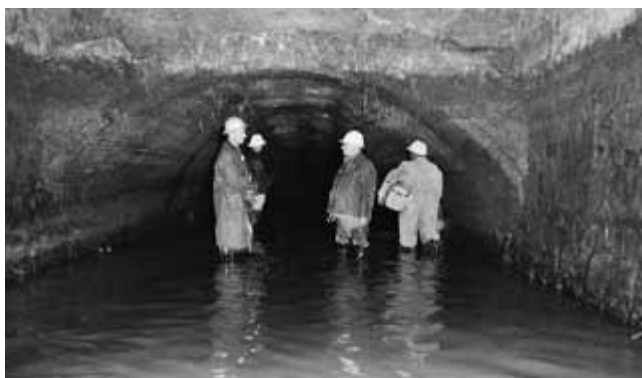
City workers inspecting 12-foot Bowery Bay sewer
