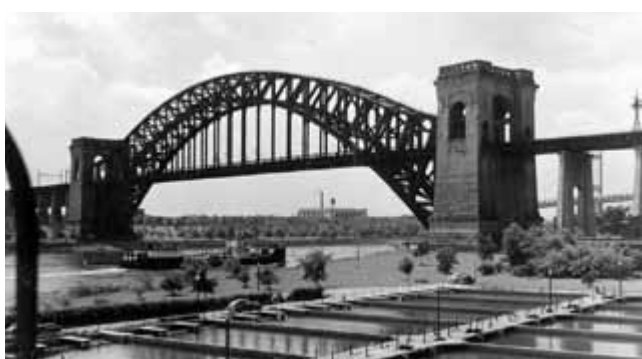
Wards Island Wastewater Treatment Plant on the East River
