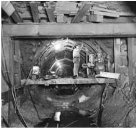
Sedgwick Avenue sewer construction (1939)
