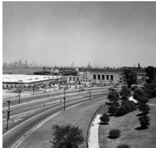
Owls Head Wastewater Treatment Plant
