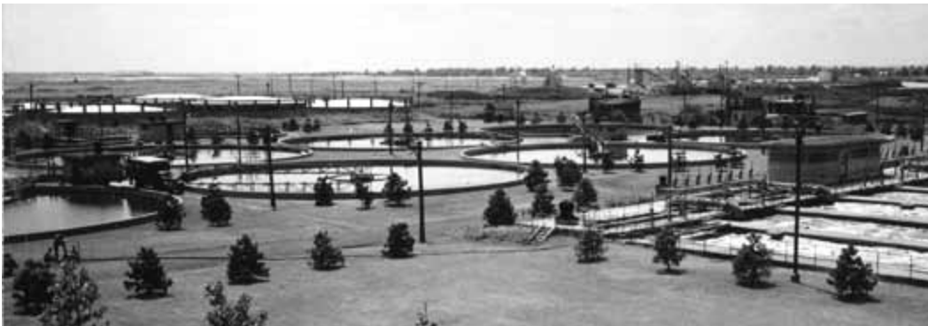
Jamaica Wastewater Treatment Plant after an upgrade
