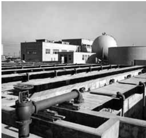
Aeration and sludge tanks at Rockaway Wastewater Treatment Plant
