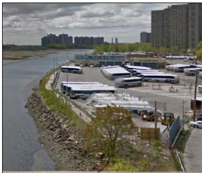
Figure 3a. Hutchinson River Shoreline (Western)
